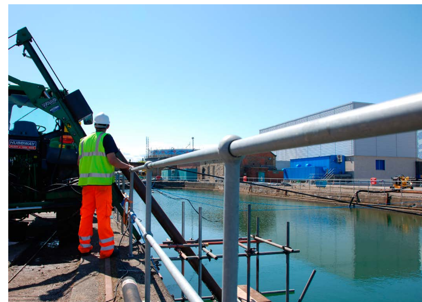
Picture 1. Post driver and piling setup.
