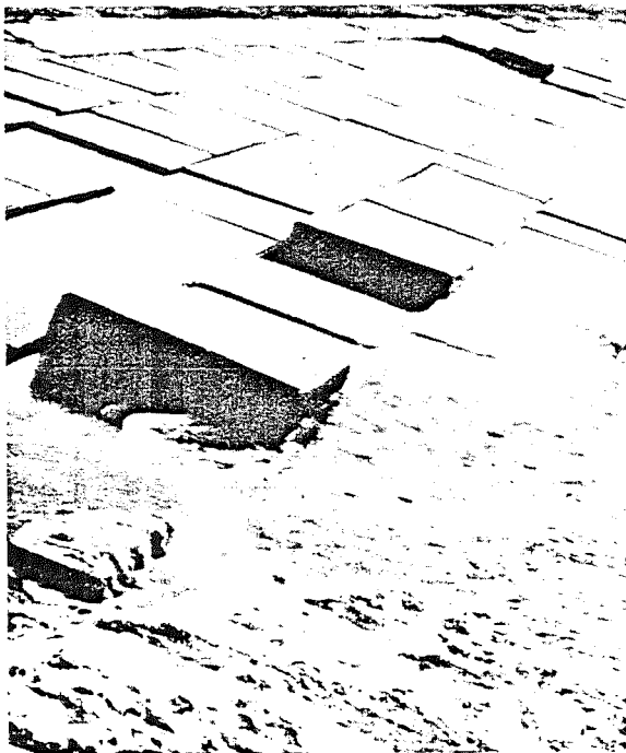
Row of units forced upwards by pressure from within the filter.
