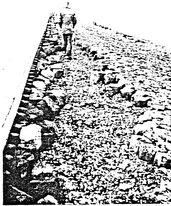
Row of units forced upwards by pressure from within the filter.
