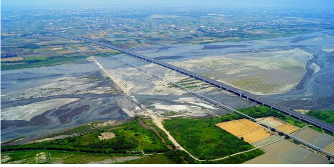
Figure 1. Photo of Zhong-sha Bridge
