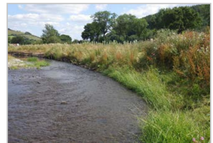
Woody products from the coppicing and pollarding staked at toe of bank immediately after the works in March 2013 (left); in June 2013 (centre) showing the first growth of the grass and live willow protection; and in June 2014 with good willow and marginal growth.
