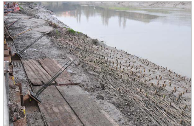
Scheme at the final stages of construction. The bottom part of the brushwood mattresses is already covered in silt. Source: Natural Resources Wales
