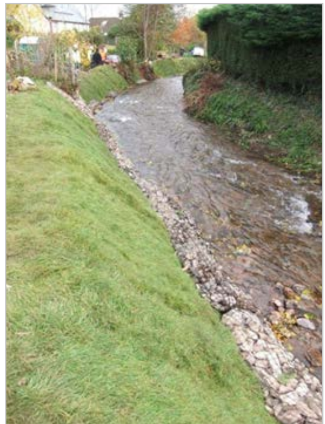
Left: Installation of toe protection (2013); Right: Completed works (2013). Source: Environment Agency
