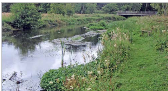
Channel narrowing caused by the wood deflectors. Source: River Restoration Centre
