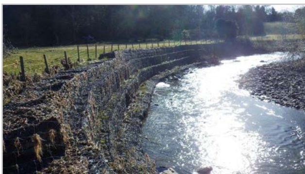
The old failing gabion baskets (left) and the new V-Max matting and (vegetated) rock rolls (right). Photo supplied by Salix Ltd
