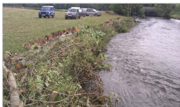
The eroded bank and footbridge downstream with strainers in place (left) and with completed protection (right). Source: Tom Dawson, Northern Habitat, Countryside Contractors
