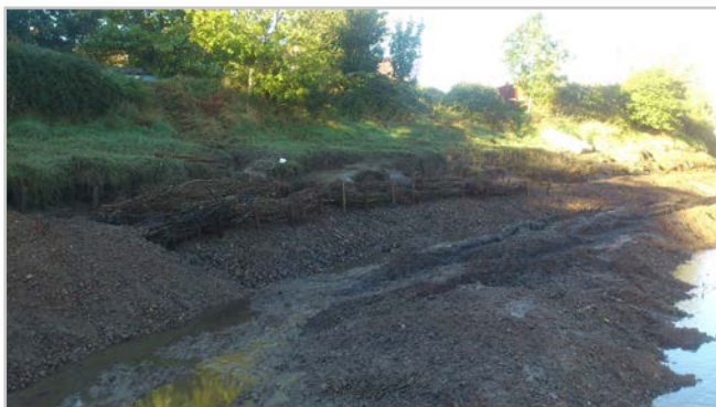
Faggots staked down above the rock roll mattresses. Source: Natural Resources Wales, 2013
