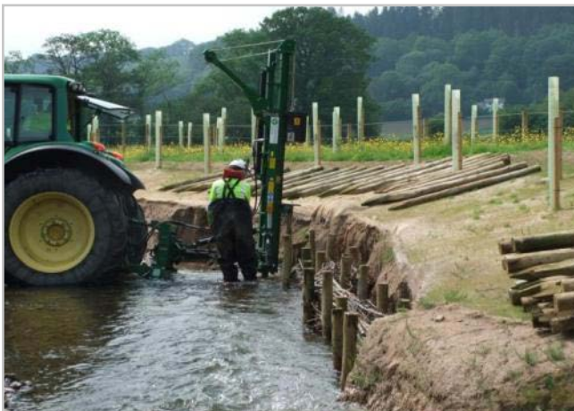
Post being driven into the bank to place the faggots. Source: Environment Agency
