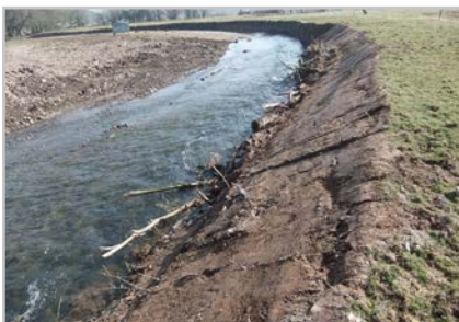
Woody products from the coppicing and pollarding staked at toe of bank immediately after the works in March 2013 (left); in June 2013 (centre) showing the first growth of the grass and live willow protection; and in June 2014 with good willow and marginal growth.
