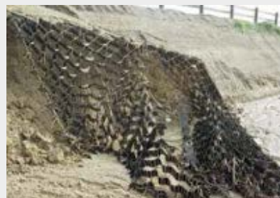
Examples: Failure of geo cell system due to inadequate connection and with improper infill (Source: Greenfix)
