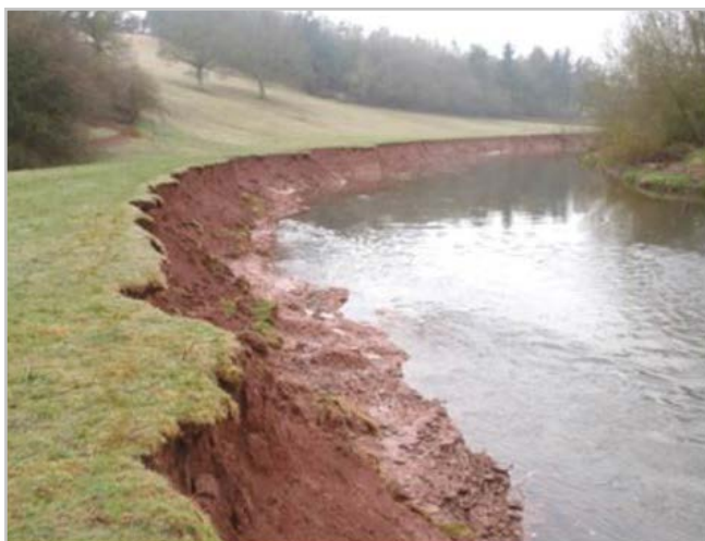
Bank erosion following the weir removal. Source: Natural Resources Wales
