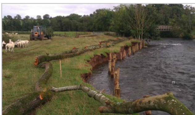
The eroded bank and footbridge downstream with strainers in place (left) and with completed protection (right). Source: Tom Dawson, Northern Habitat, Countryside Contractors
