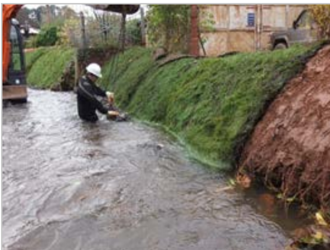
Left: Installation of toe protection (2013); Right: Completed works (2013). Source: Environment Agency
