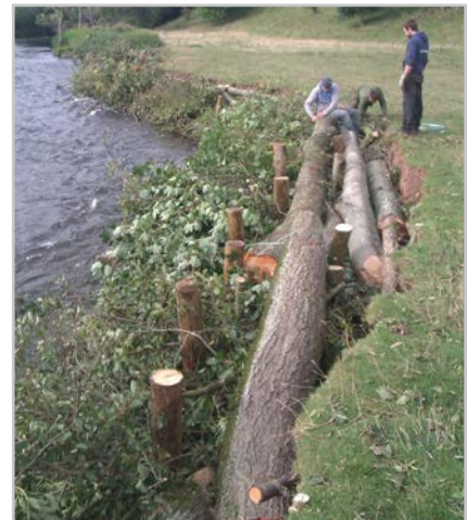
First layer of brush mattresses on top of footer logs (left) and second layer of brush mattresses and top logs (right), looking upstream.
