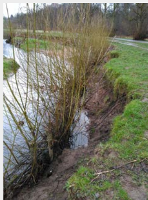
Examples: (Left) Example of loss of material behind rocks due to lack of filter (Source: NRW), (Right) Example of loss of material behind willow spiling due to lack of filter (Source: RRC)
