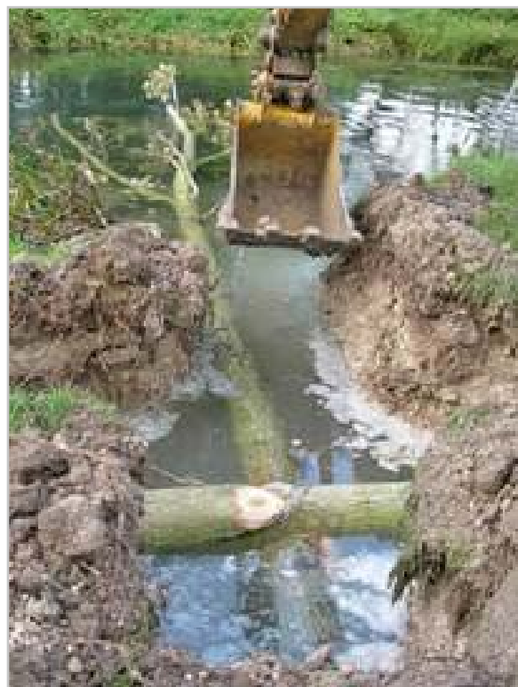
The 'crucifix' as it is placed in the trench before being backfilled. Source: Natural England
