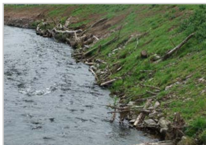
Woody products from the coppicing and pollarding staked at toe of bank immediately after the works in March 2013 (left); in June 2013 (centre) showing the first growth of the grass and live willow protection; and in June 2014 with good willow and marginal growth.
