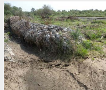
Examples: Failure of vegetated gabions due to development of scour and outflanking (Source: HR Wallingford)
