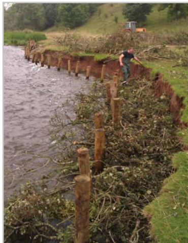
First layer of brush mattresses on top of footer logs (left) and second layer of brush mattresses and top logs (right), looking upstream.
