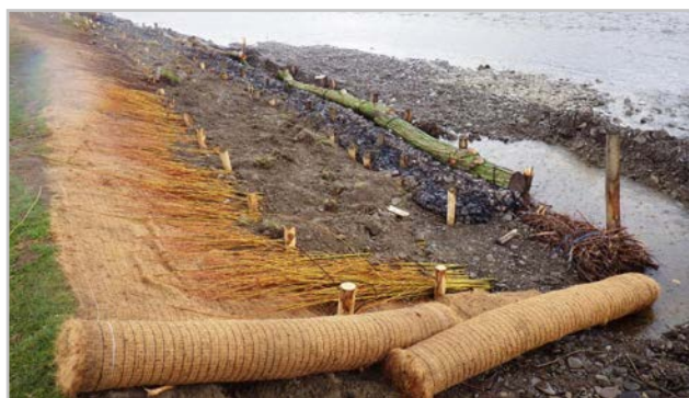
Part of the protection: coir matting, stakes, willow sprouts (bank) and rock rolls, logs, faggots staked down (toe). Photo supplied by Salix Ltd
