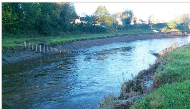
Wooden pile groynes diverting the flow away from the banks. Source: Natural Resources Wales, 2013
