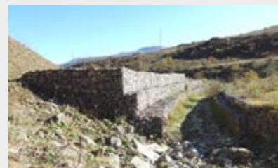
Examples: Upstream edge of gabions protection without transition (Source: HR Wallingford)
