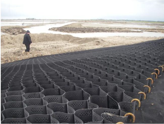
Photo 15 Cellular mattress prior to gravel filling
