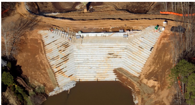
Figure 1. Y-16 Dam RCC Protection during Construction.
