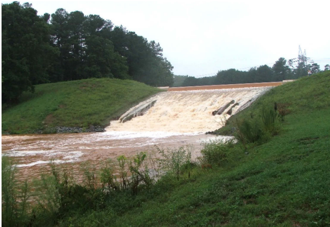
Figure 8. Y-16 Dam During Overtopping Event.
