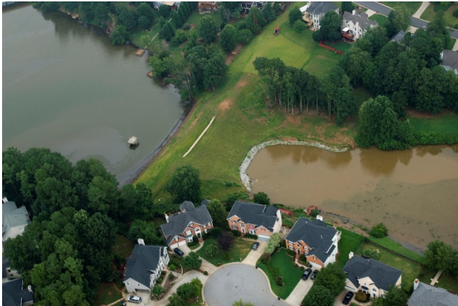
Figure 8. Y-16 Dam During Overtopping Event.
