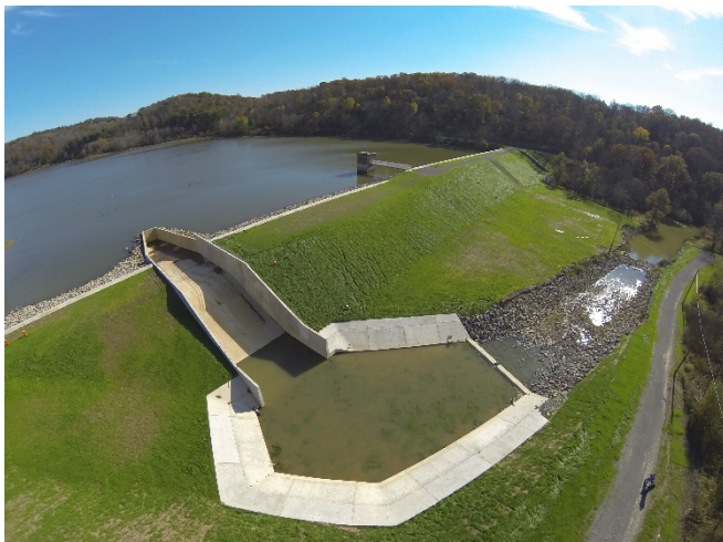
Figure 2. Lake Oneida Dam with Buried RCC Protection.
