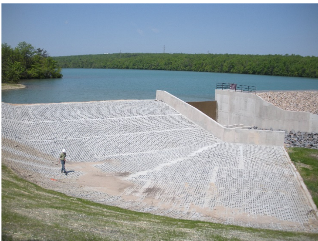
Figure 5. Mount Laurel Dam with ACB Armored Spillway.
