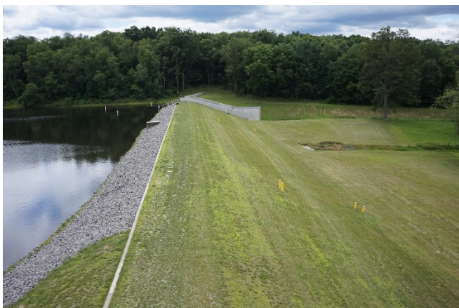
Figure 6. Glade Run Lake Dam with ACB Armored Slope.
