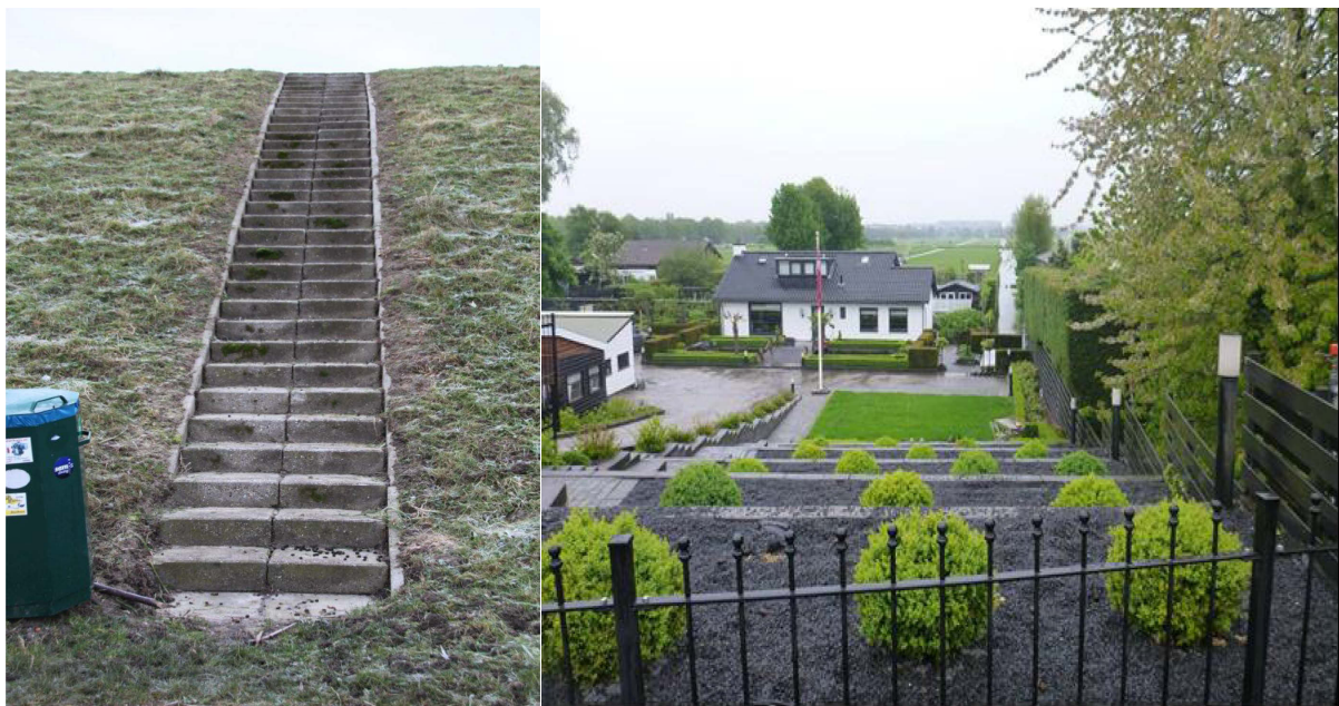
Figure 2.2 On the left: Area directly adjacent to the stairs has no grass, nor roots and is called patchy grass; Tholen, Section 2, Stair (before testing). On the right: typical layout of a Dutch garden on the landward slope of a river dike
