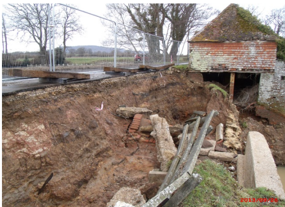
Figure 5. Erosion behaviour at a small dam affected by soil type and road cover (appears dominant) and transitions between soil and various structures (Photo: Alan Brown)
