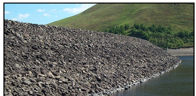
Figure 5: Rock armoured (asphaltic grouted rip-rap) embankment dam (Megget).
