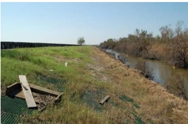
Figure 4. The undamaged levee after the stormwater receded. The project's success started a 10 year USACE research program to understand HPTRM technology.
