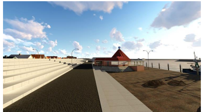
Figure 1. Artist impression of design of primary flood defence with stair shaped revetment at Den Oever, The Netherlands
