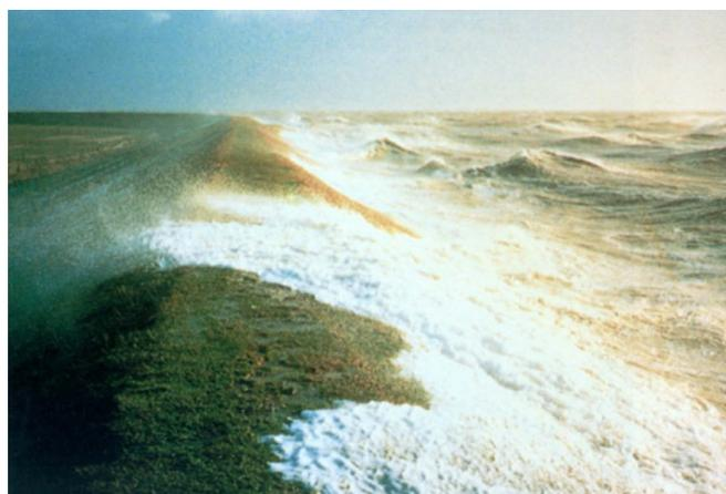
Figure 1. Wave overtopping of a grass covered dike at Hartlepool, UK. Picture courtesy: HR Wallingford.
