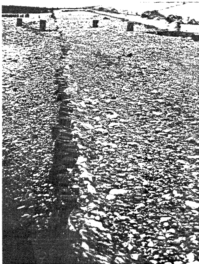
18 Foreshore replenishment showing filter fabric to deter leaching
