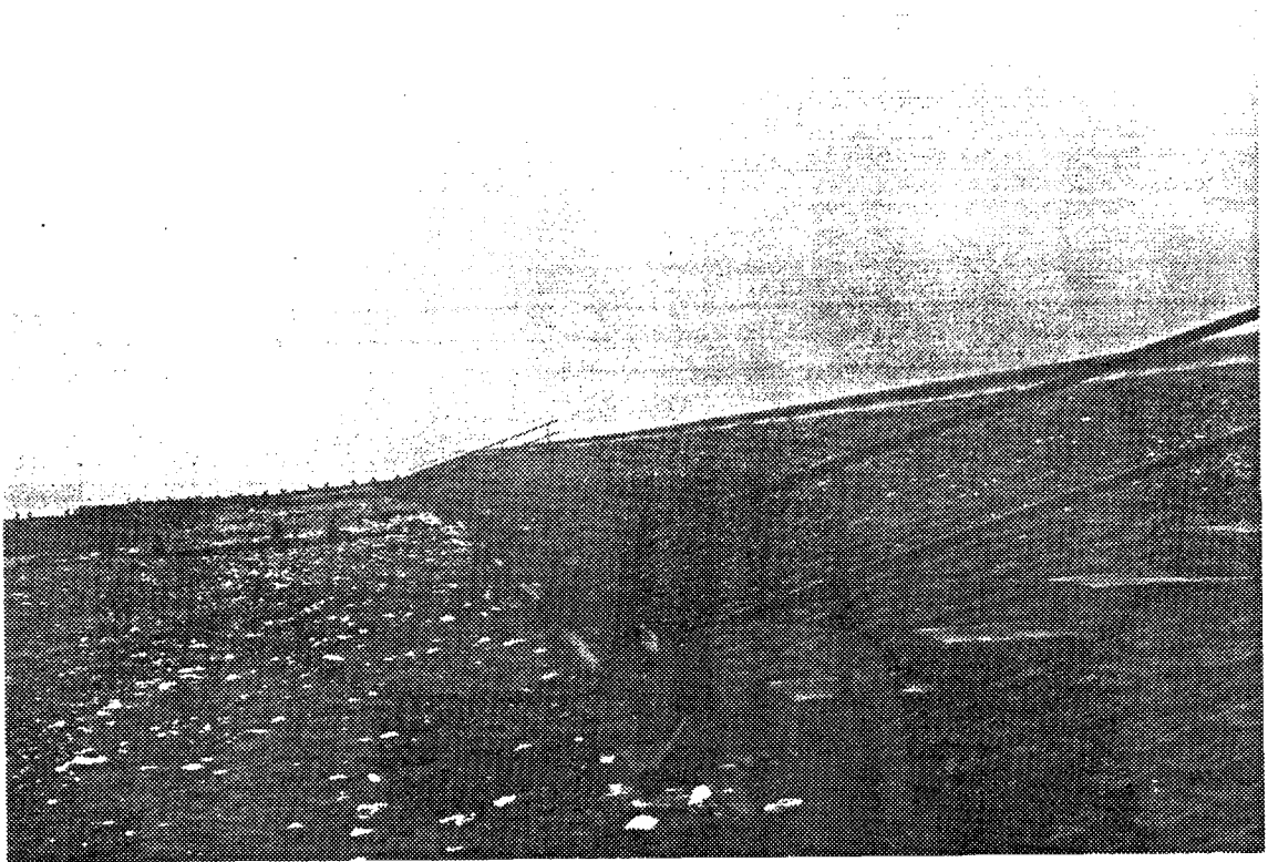
9 Section 3 (Petriflex) showing swash line
