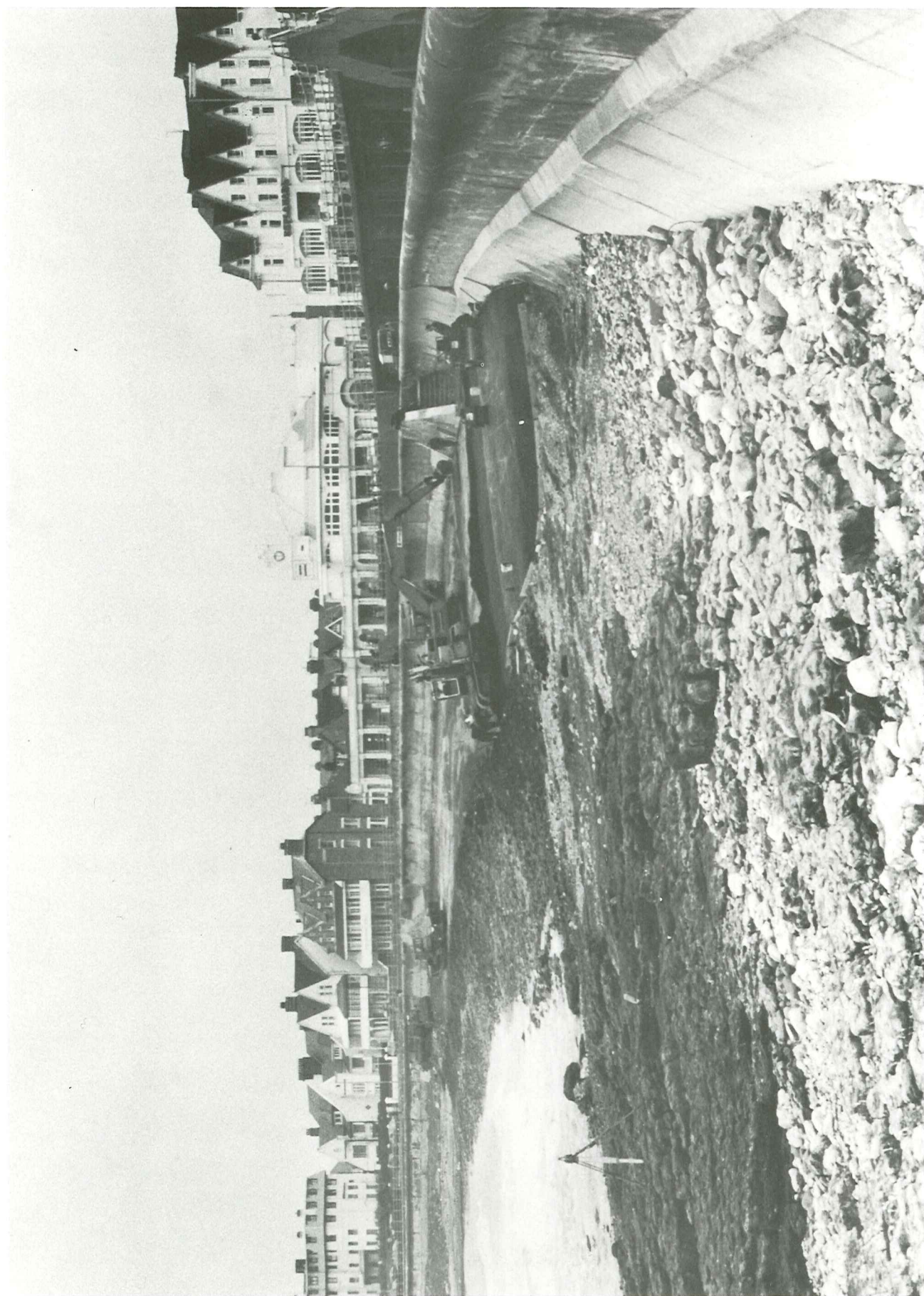
14. Asphaltic revetment under construction - Porthcawl, Glam
