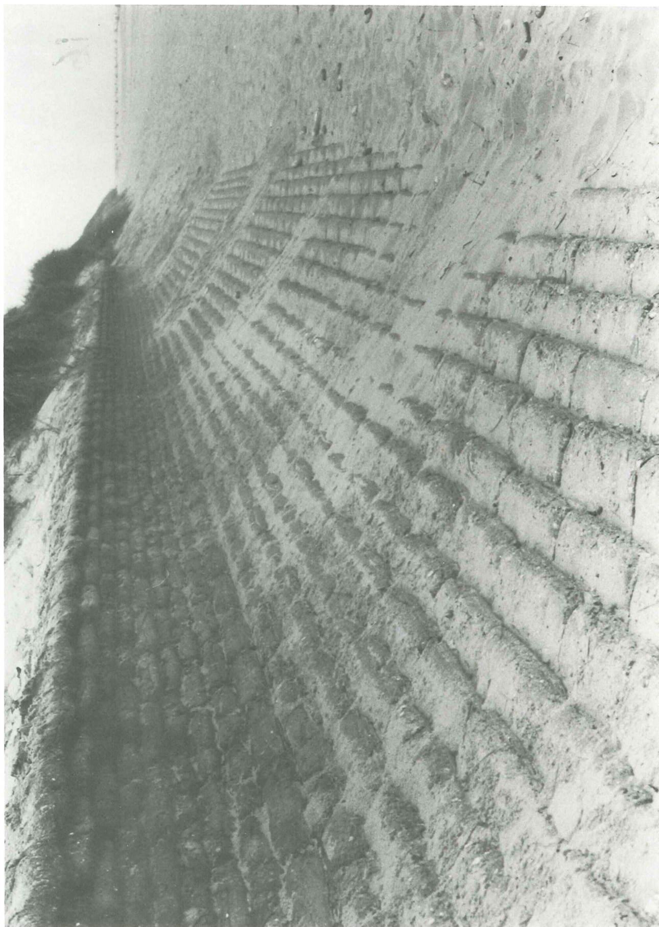
17. Sand-cement bag revetment - Eccles, Norfolk
