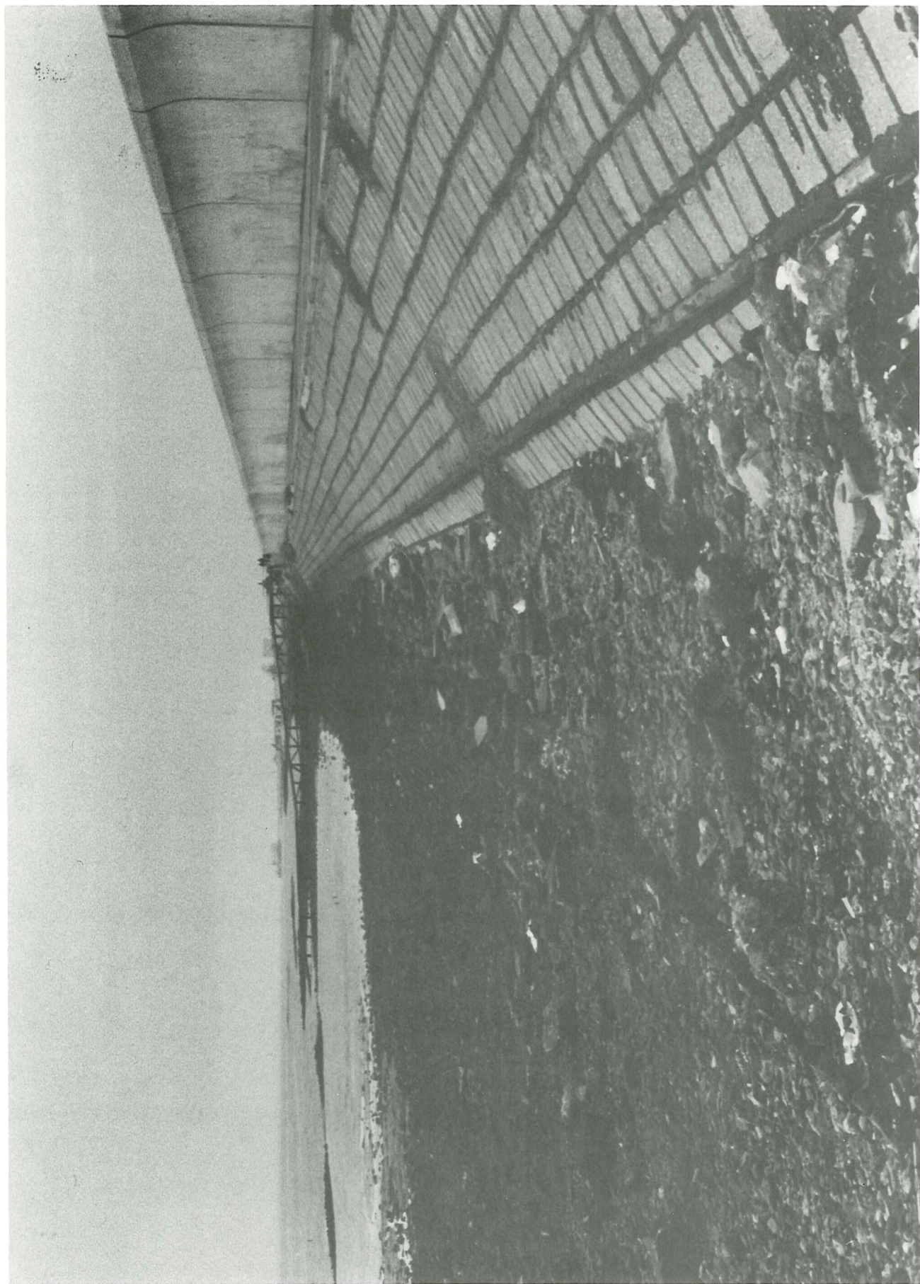
4. Asphalt grouted blocks - Canvey Island, Essex
