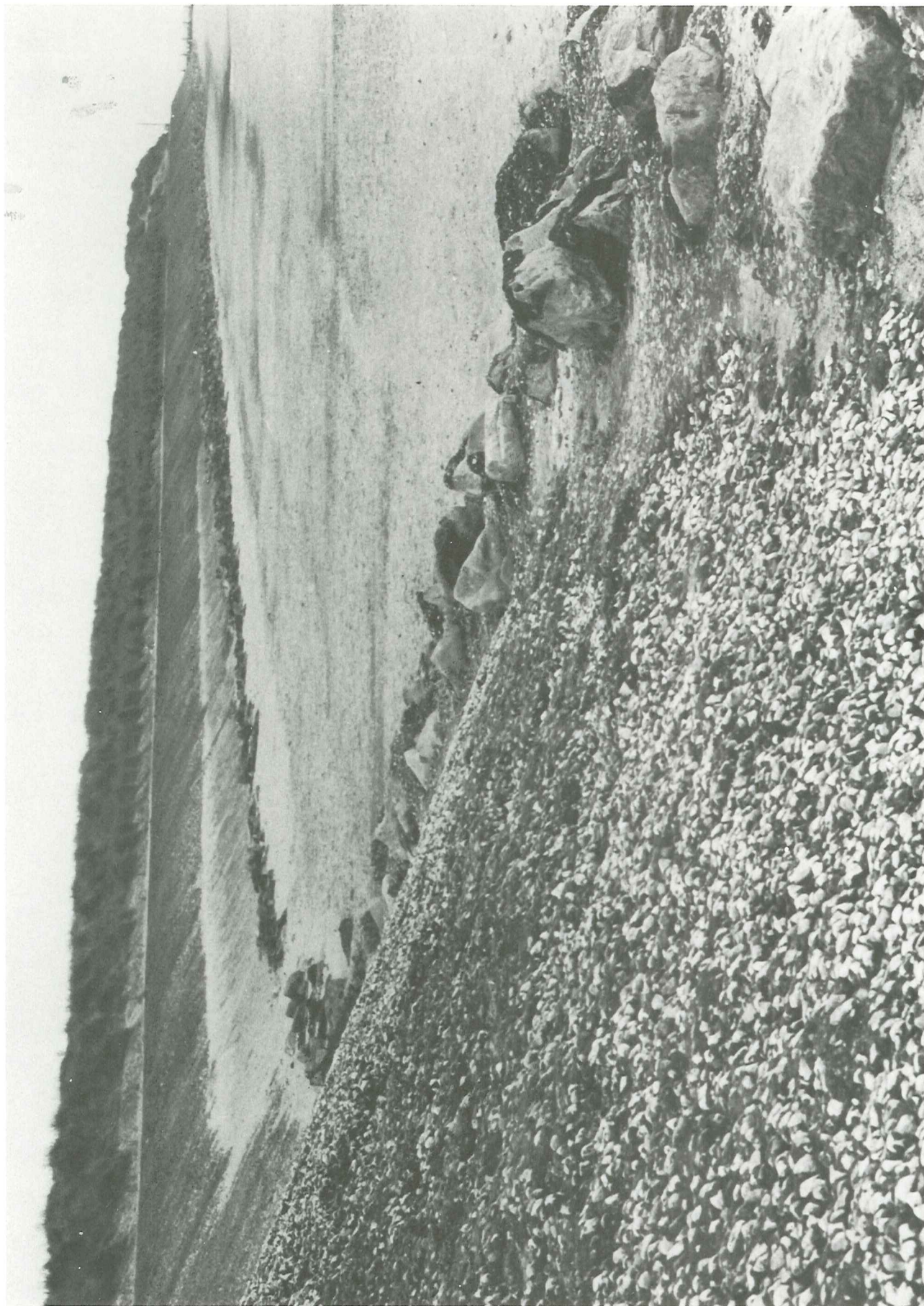
12. Asphaltic revetment - Caister, Norfolk
