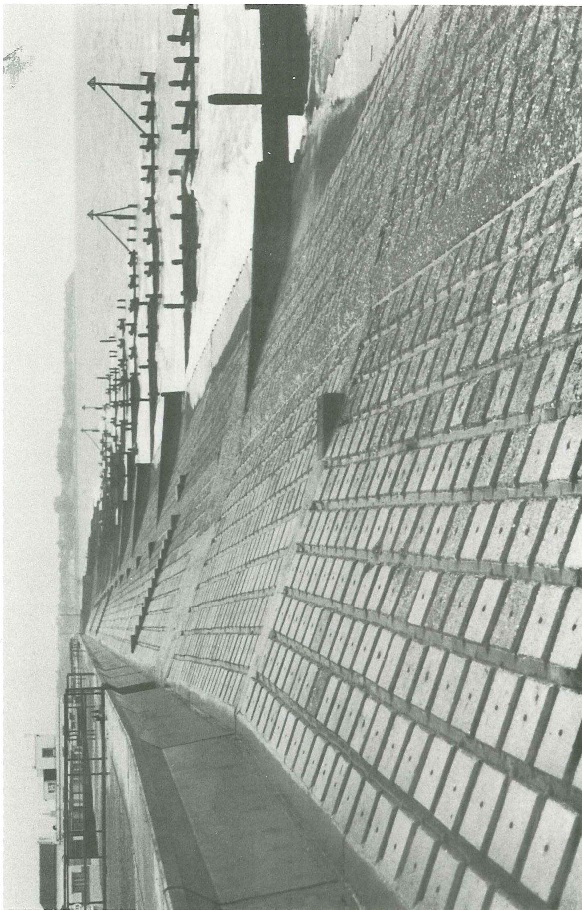
5. Asphalt grouted blocks - Landguard Point, Felixstowe, Suffolk
