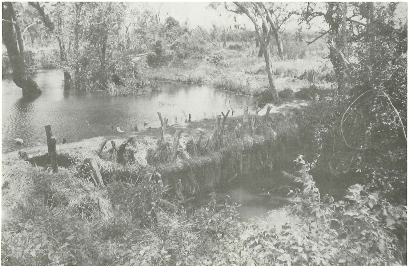
PLATE 18 Weir across stream to divert drainage water for re-use
