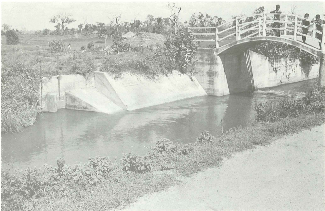
PLATE 9 Drop structure at 2 m 27 ch on Stage II Branch Channel 1 with offtake to Tract 6
