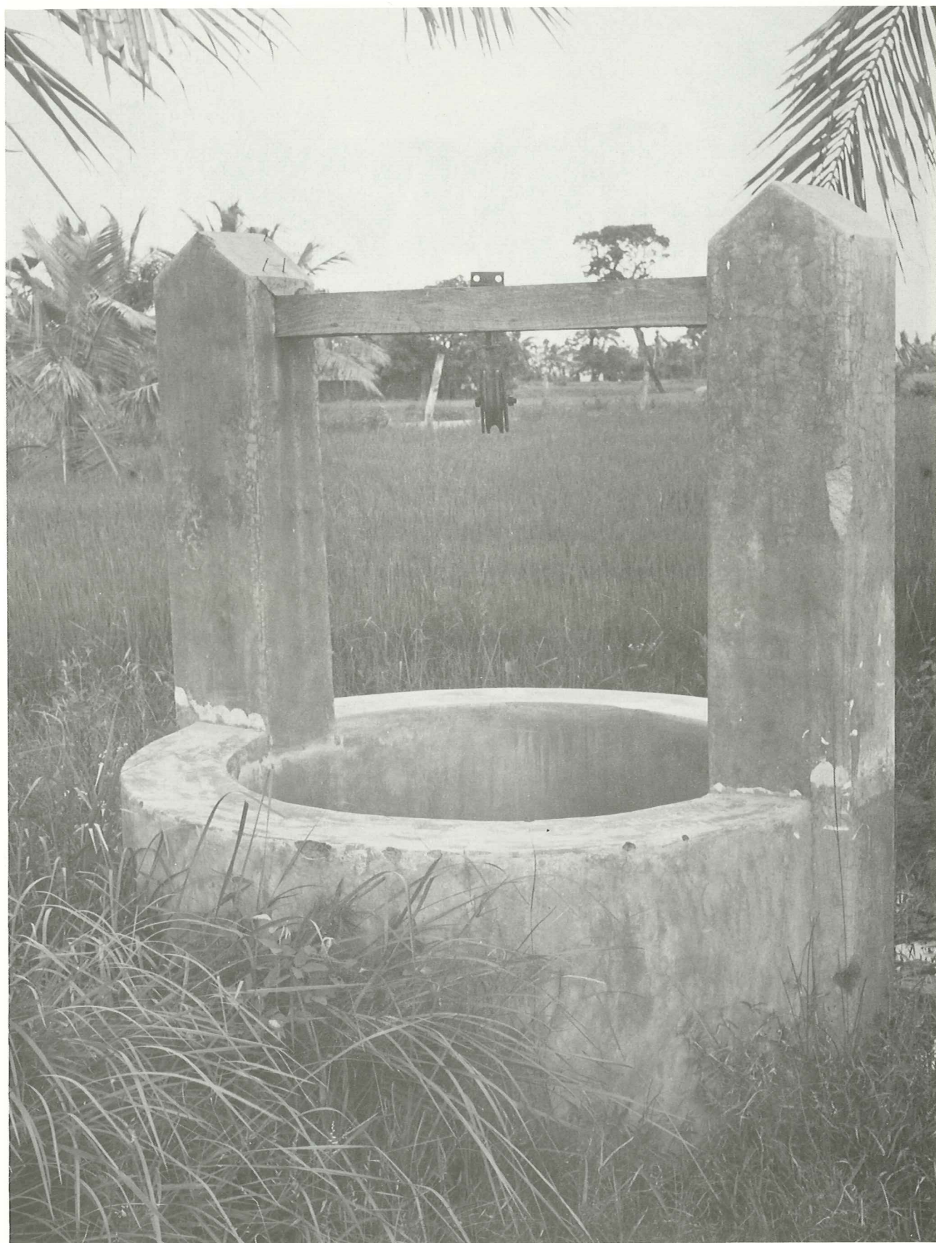
PLATE 19 Groundwater Observation Well
