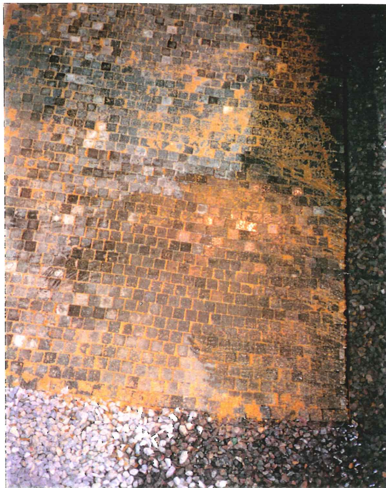
Plate 8 Concrete block on bank with slope 1:2.5. Staggered
