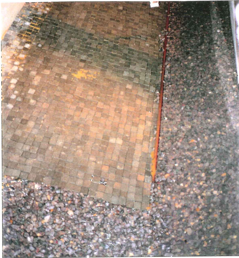
Plate 7 Concrete blocks on bank with slope 1:2
