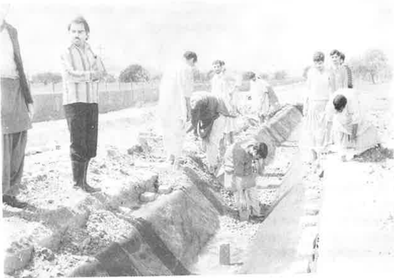
Photo 6. Taurus rubber sheet spread in experimental water channel section prior to providing soil cover Naiz Beg Research Station, Lahore.
