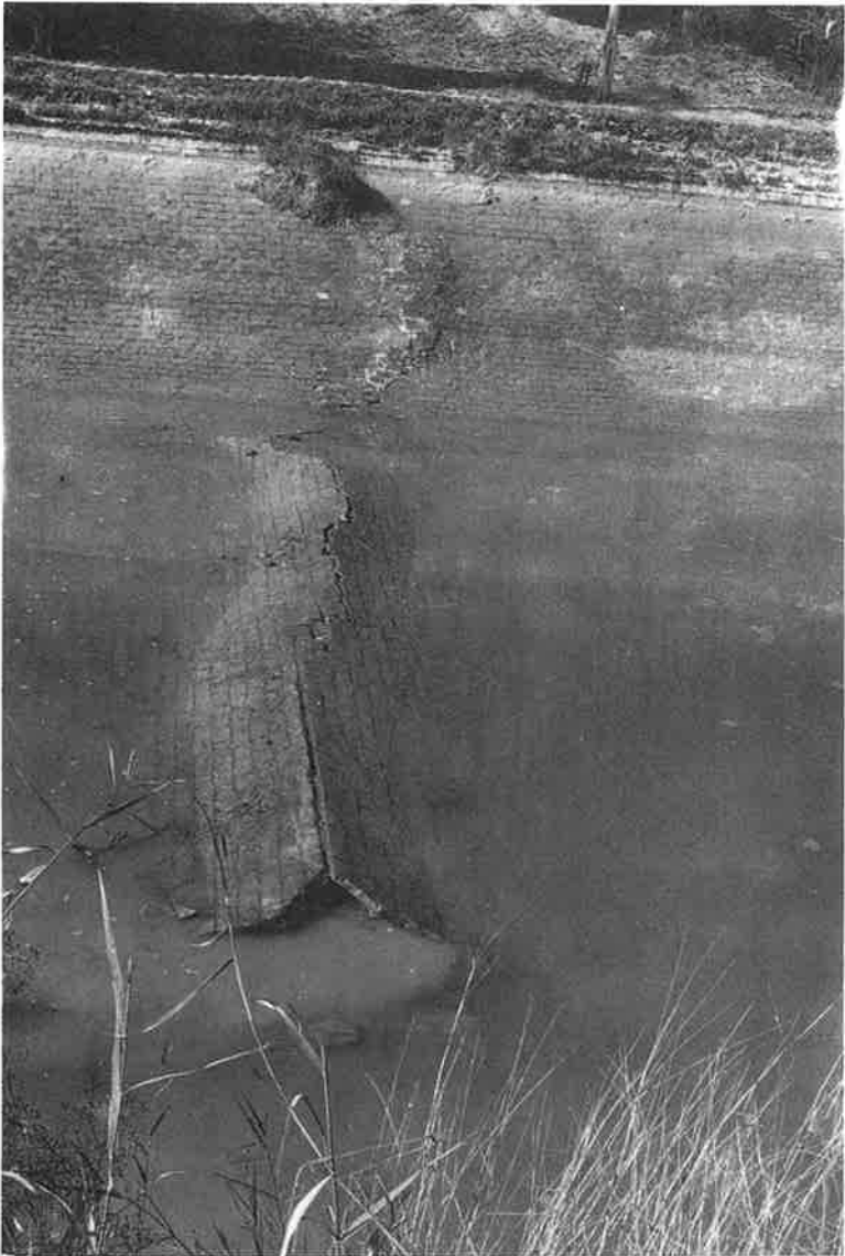
Figure 4A. Lined Bed of Haveli Canal Lift-up by Water Pressure.
