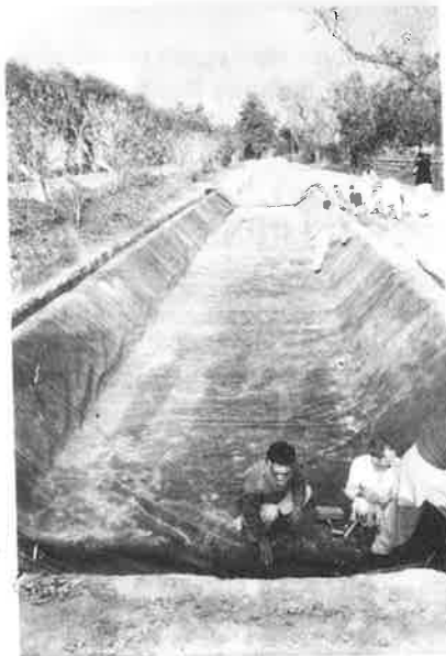
Photo 7. Mizu rubber sheet spread in experimental channel and anchor trenches at Nandipur Research Station, Gujranwala.
