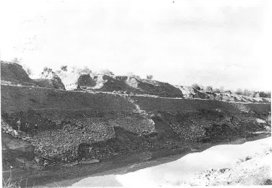
Figure 4B. Specimen of Damaged Lining of Thal Main Line Upper.
