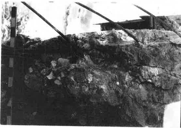
Figure 5. Right Bier of East Spillways of Huai Rou Reservoir.
