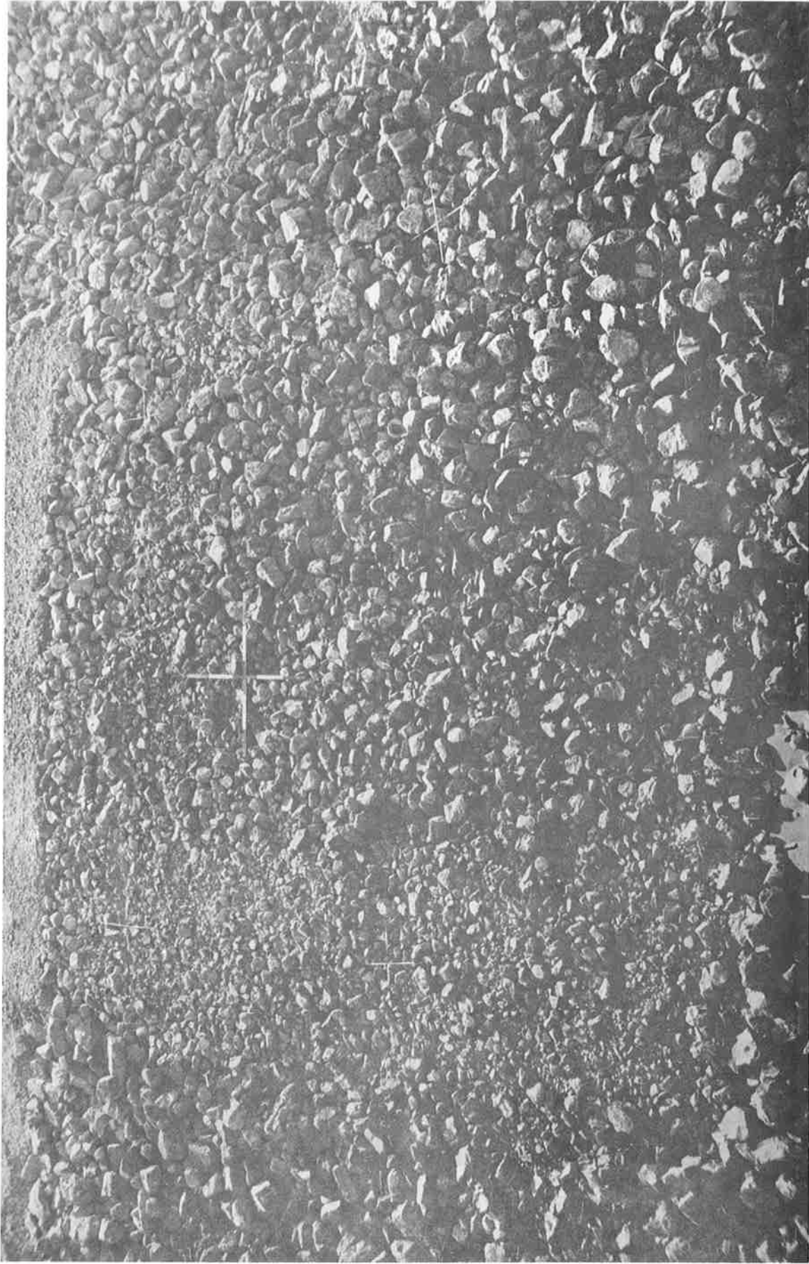
Plate 1 Field riprap panels 1-4
