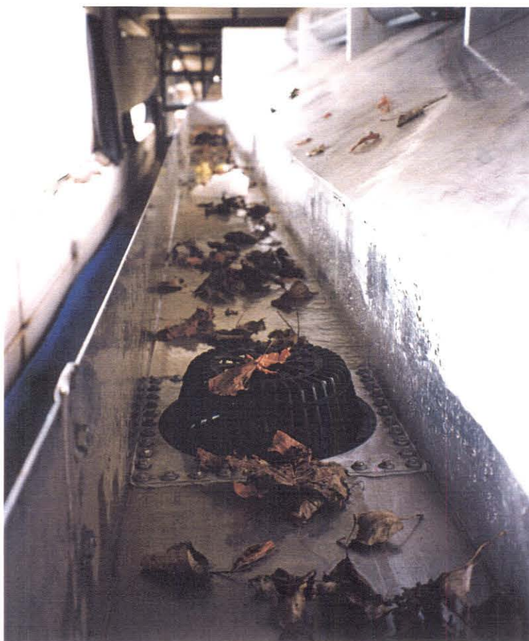
Plate 14 Test with debris in the gutter (beginning of test)
