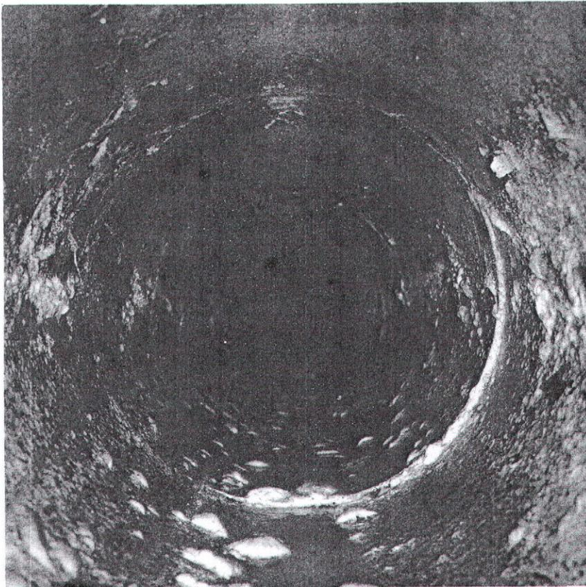
**Plate 7** Roughness of composite surface (pipe-full)  $k_c = 3.2\text{mm}$
