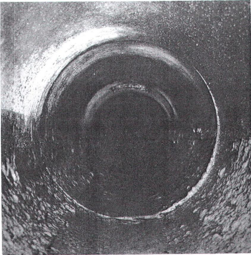
**Plate 6** Roughness of composite surface (pipe-full)  $k_c = 1.8\text{mm}$
