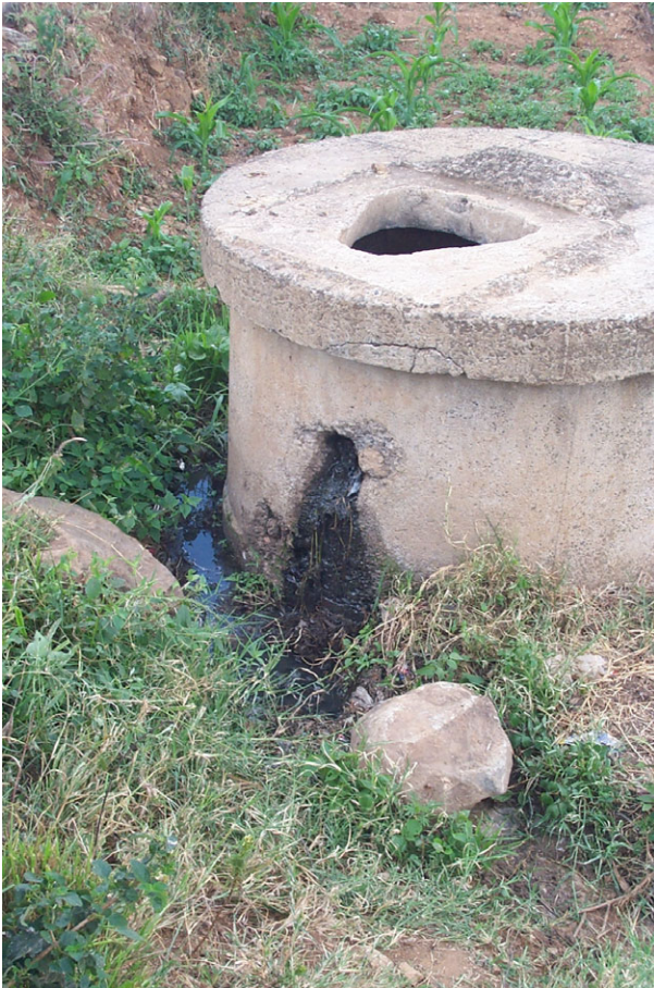
Figure 7 Broken manhole at Maili Saba
