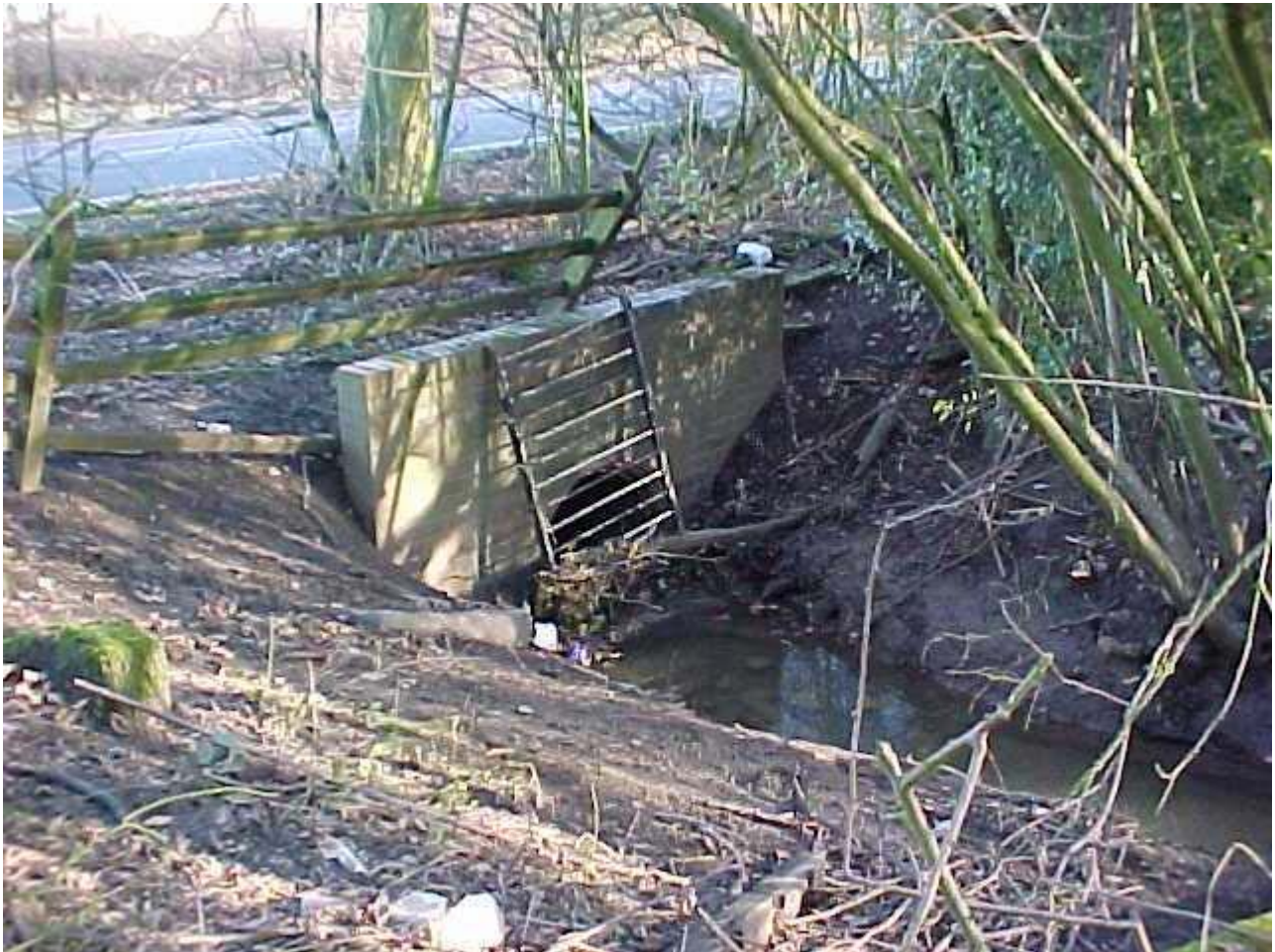
Plate 7 Upstream side of culvert beneath A5 at Merevale
