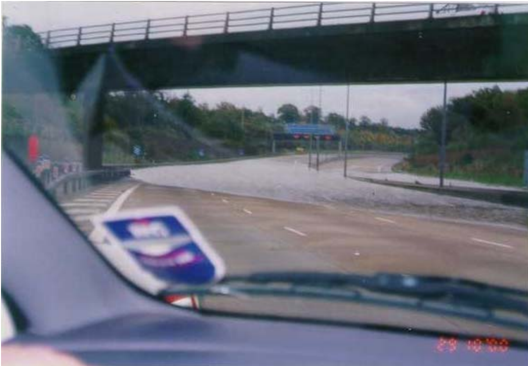
Plate 1 Flooding on the M25 at Junction 9 on 30/11/00 (NB not 29/11/00 as shown)
