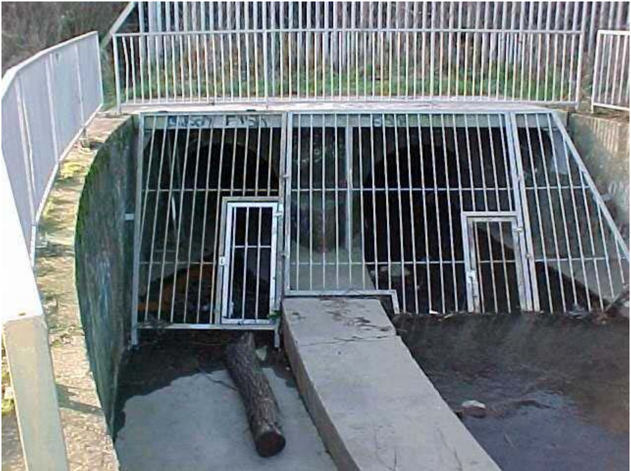
Plate 8 Upstream side of culvert beneath A5 at Kettlebrook
