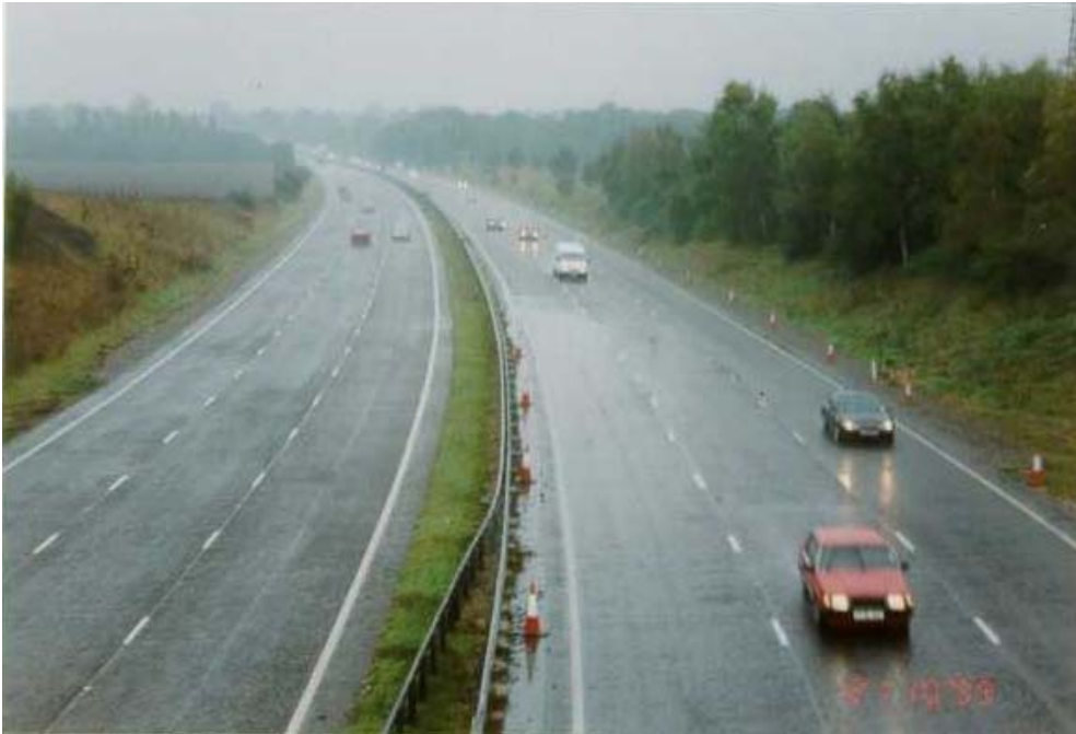
Plate 5 Ponding on A3 near Junction with A247 due to lack of camber at transition
