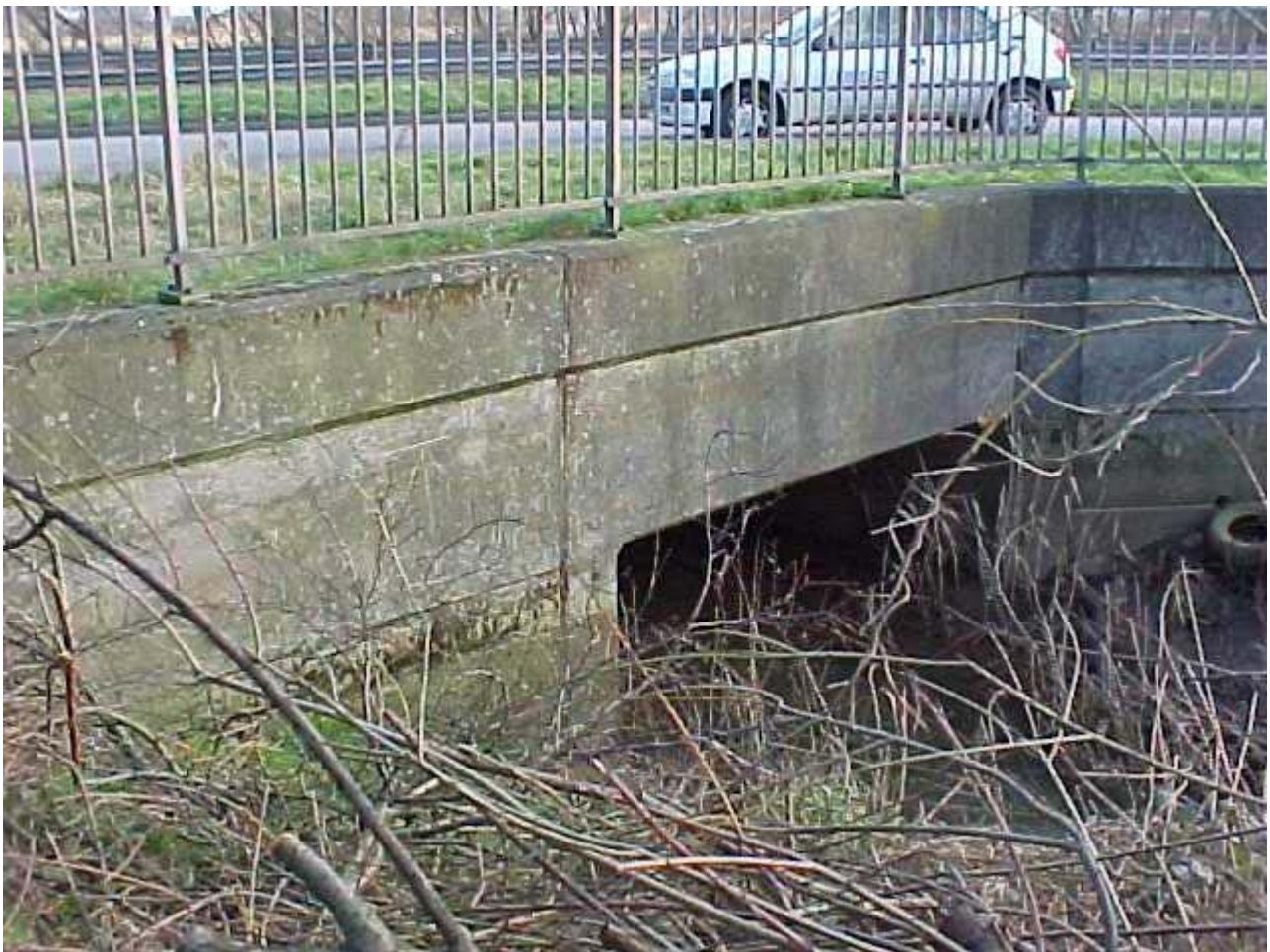
Plate 9 Culvert beneath A38 at Branston
