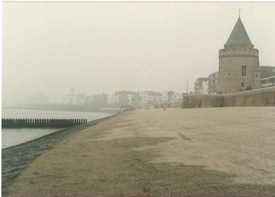
Plate 1 Vlissingen. Brick sea wall protected by a wide asphaltic concrete revetment.
