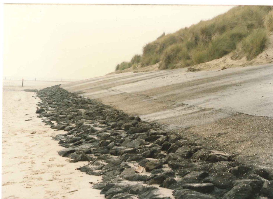
Plate 4 Westenschouwen. Asphaltic protection to toe of dunes.
