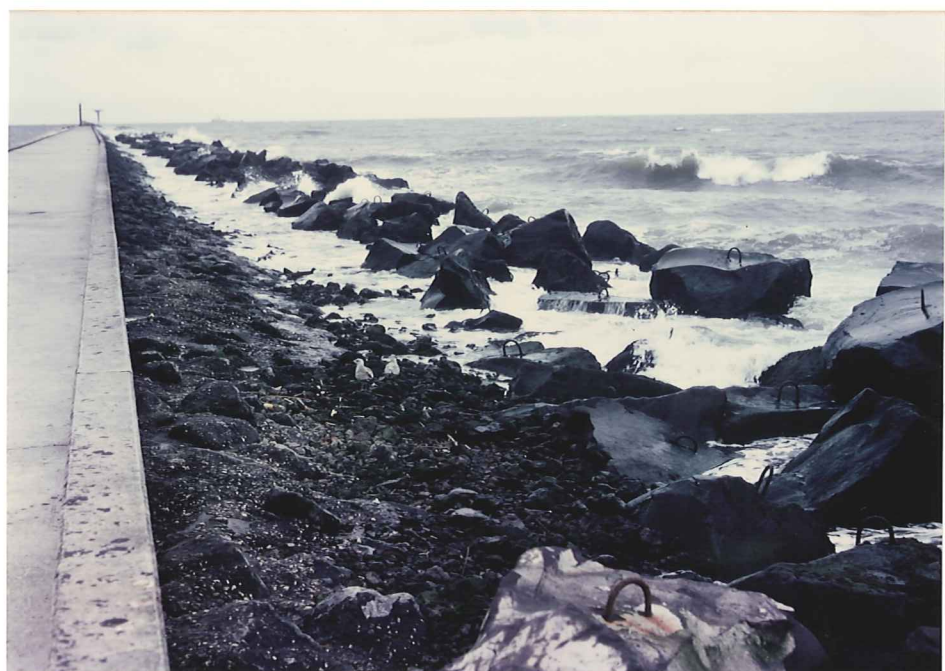
Plate 10 Hoek van Holland. North breakwater protected by asphalt grout and by a reef of large rocks.
