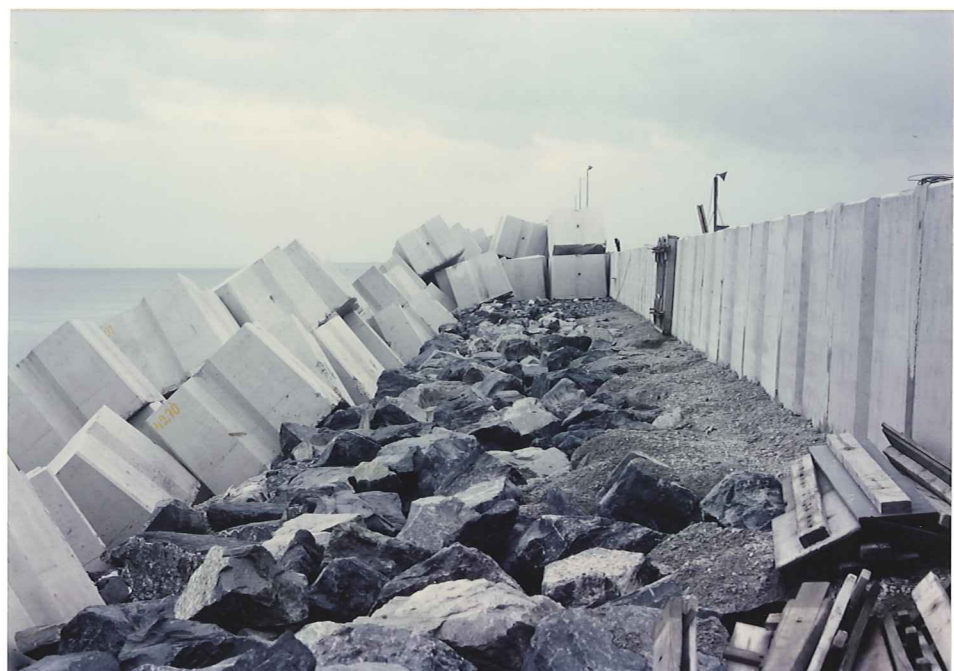
Plate 14 Zeebrugge. Concrete armour units protecting the new south breakwater.
