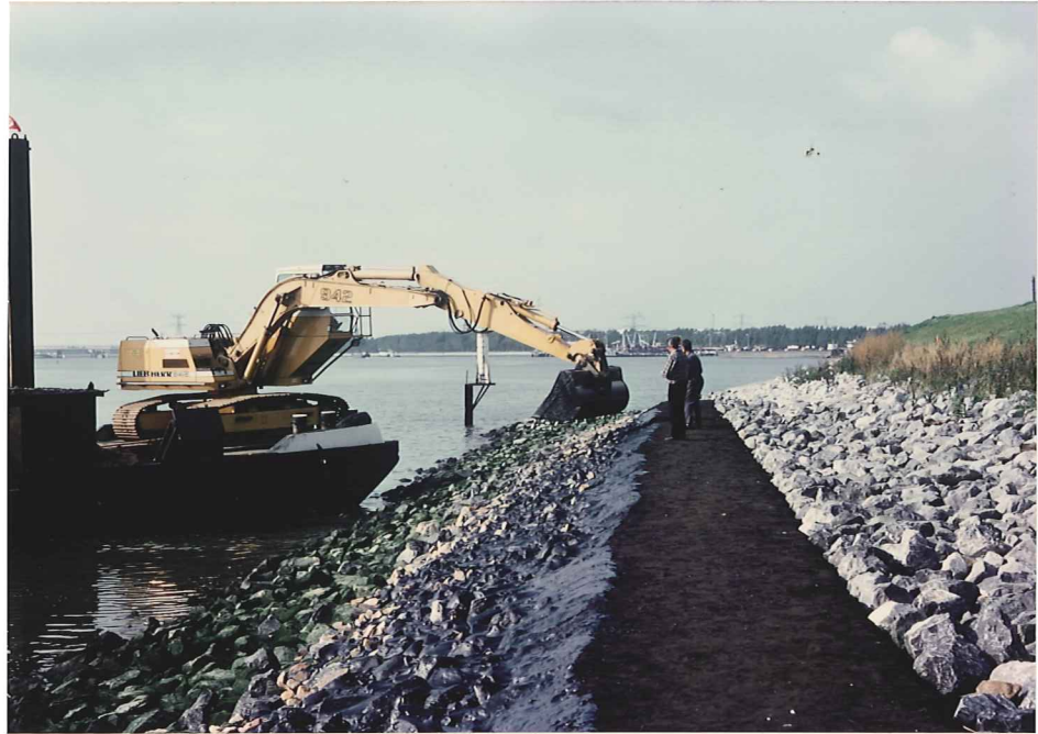
Plate 9 Rotterdam Waterway. Small scale bank improvements using asphalt grout and sand asphalt.
