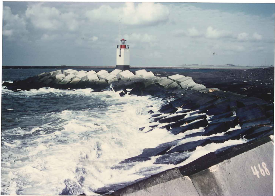
Plate 13 Ijmuiden. Spur breakwater armoured with large concrete armour units.
