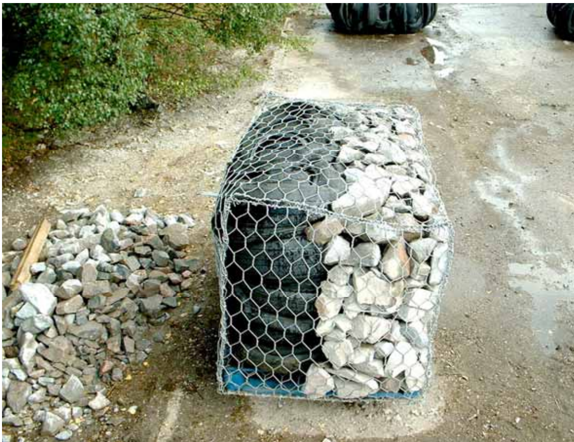
Figure 5.39 Tyre bale as rear fill for gabion box (courtesy Northern Tyre Recycling)
