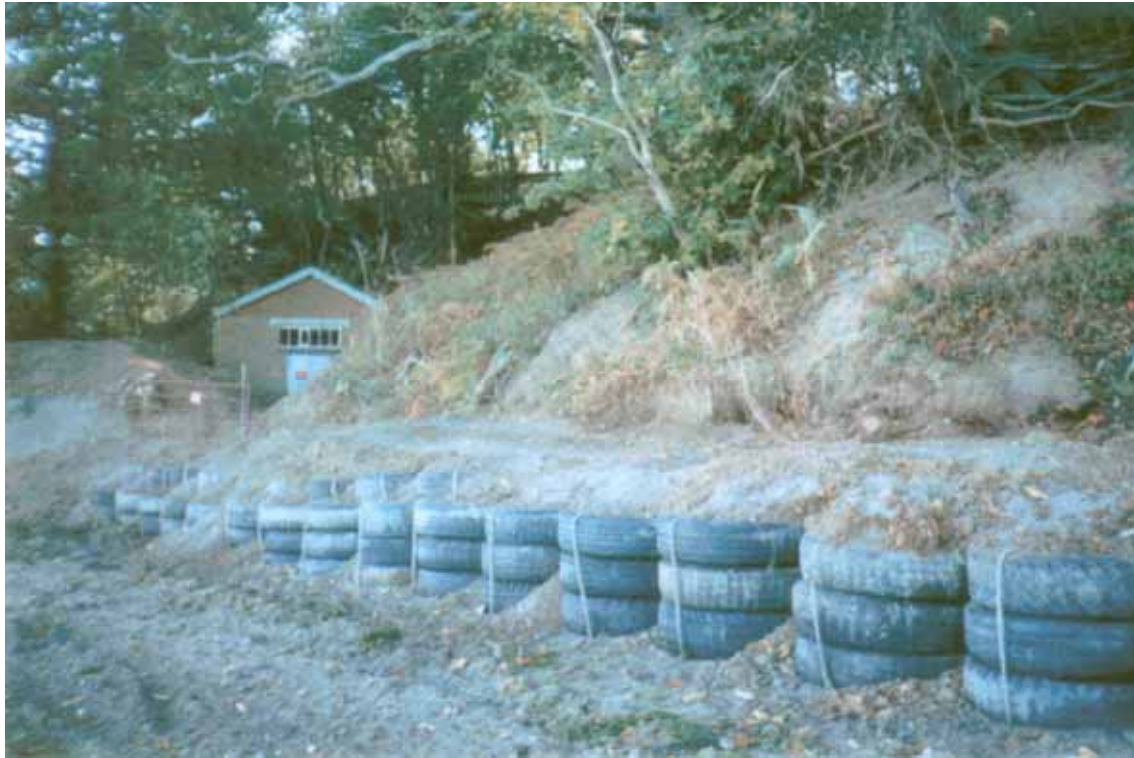
Figure 5.7 The Copperas Wood defence soon after construction (courtesy of Sorrell Flood Protection)
