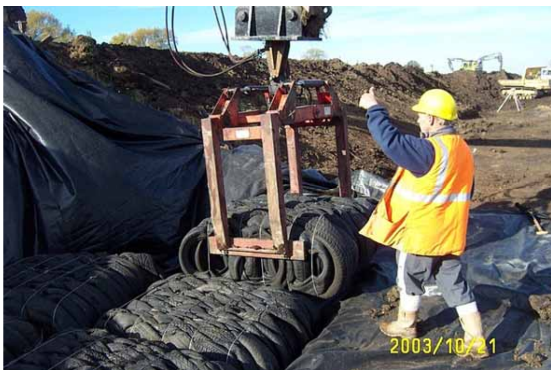
Figure 4.7 Placement of tyre bale into structure using a pallet grab attachment (courtesy Environment Agency)
