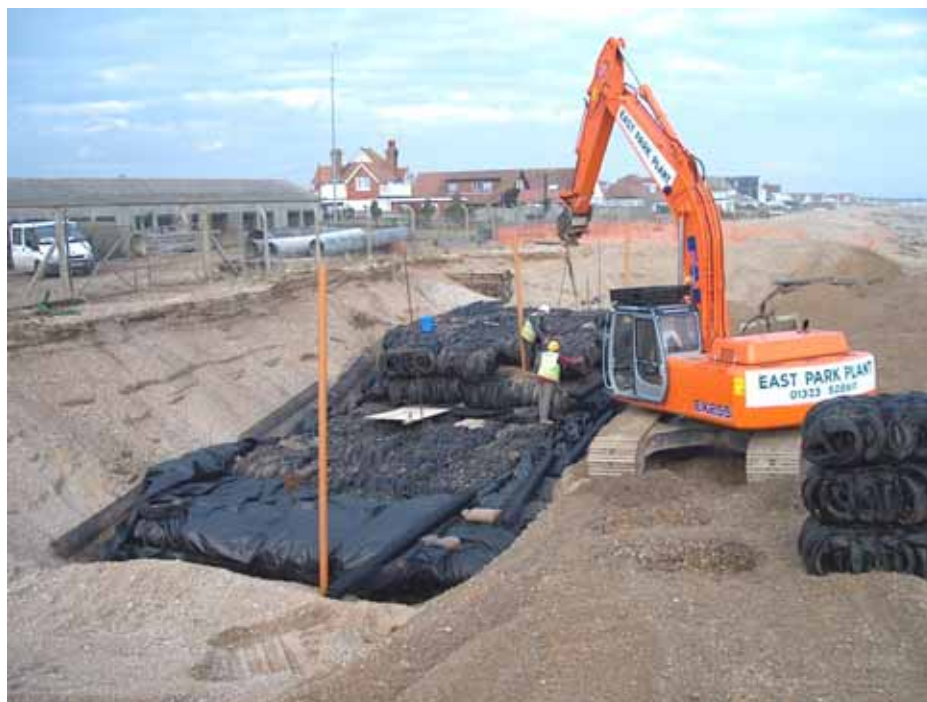
Figure A8.12 Construction of the tyre bale block in Pevensey Beach (Courtesy of PCDL)
