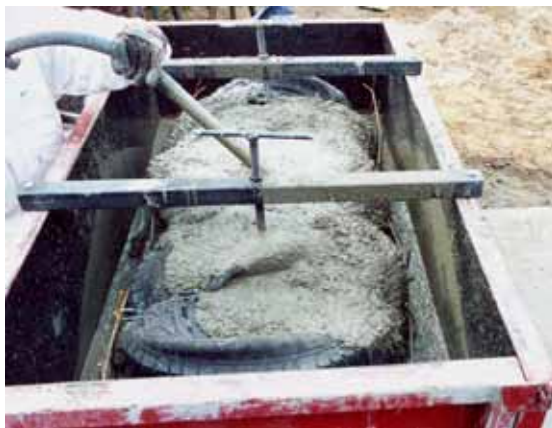
Figure 5.40 Concrete being poured around tyre bale into block cast (courtesy Northern Tyre recycling)
