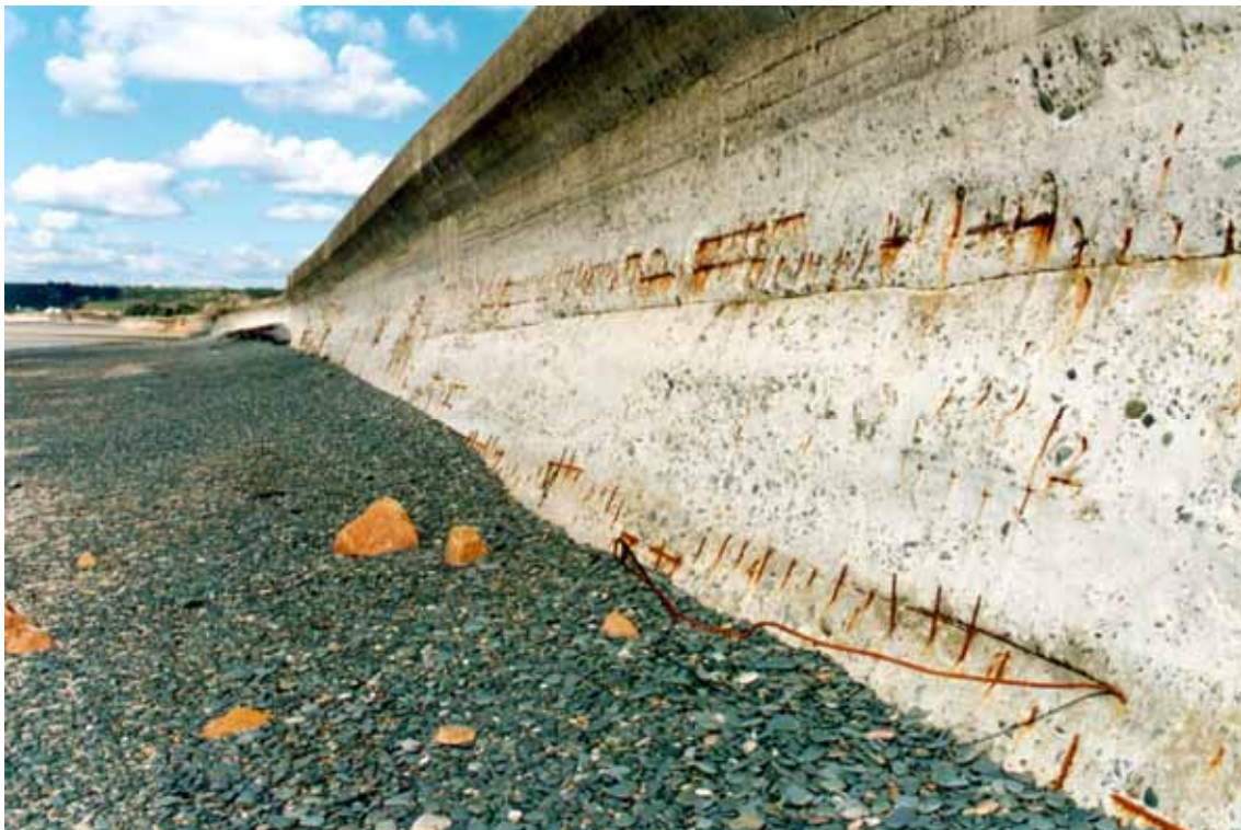
Figure 3.2 An example of hydrodynamic abrasion exposing steel reinforcement in a concrete seawall
