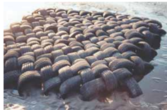
Figure 5.14 RINGtech® erosion protection matting and hollow bodies (courtesy RINGtech®)
