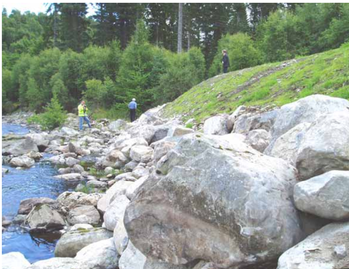
Figure 5.35 Rock armour placed for bank toe protection
