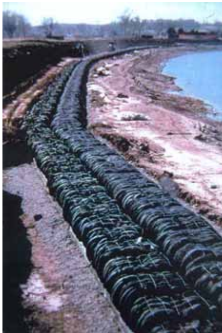
Figure 5.26 Bank stabilisation of the Pecos River in New Mexico using tyre bales (courtesy Encore Systems)
