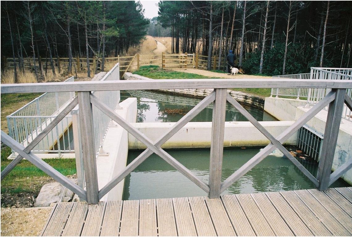
Figure 6.14 Outfall infrastructure at Elvetham Heath, Hampshire
