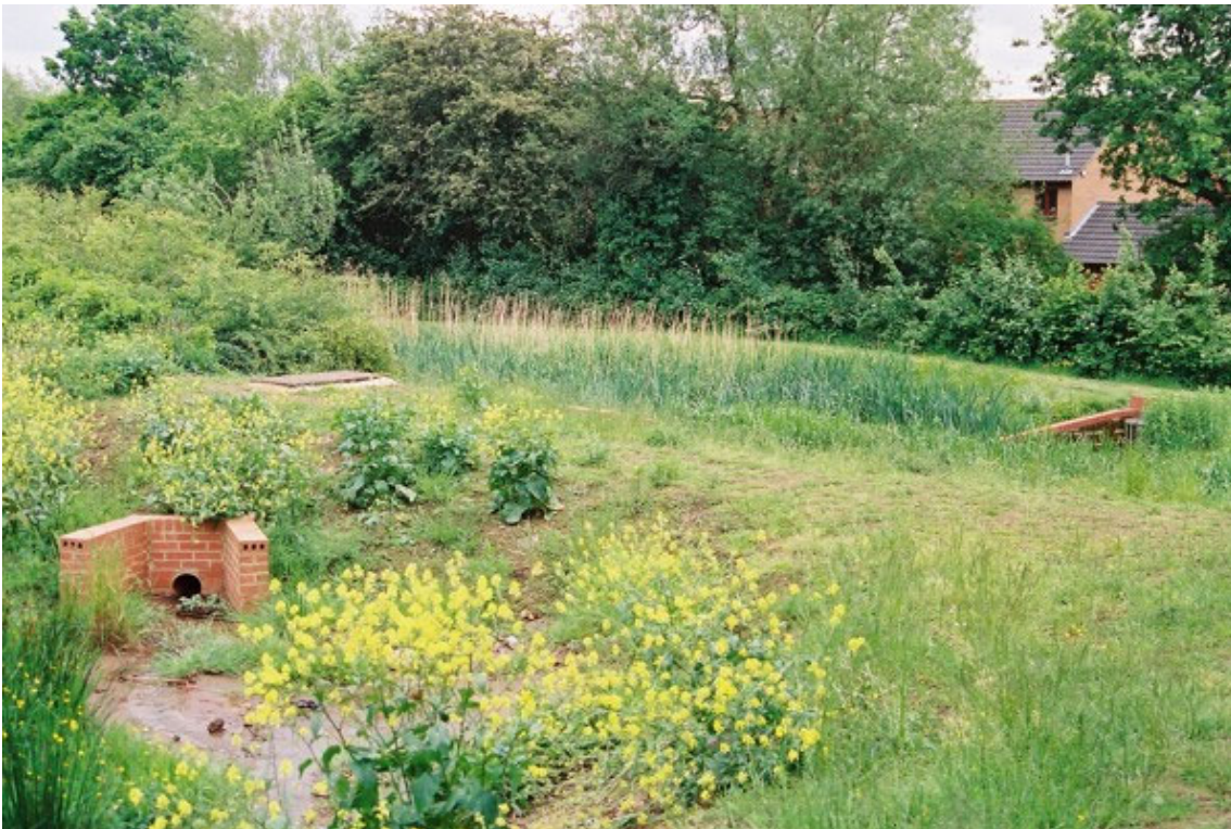
Figure 6.15 Outfall infrastructure, North Common, Bristol
