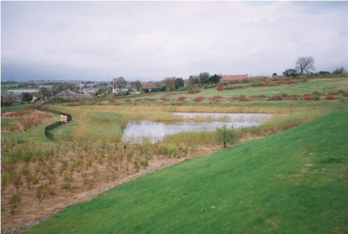
Figure 6.13 Retention pond with high density vegetation, DEX site, Dunfermline
