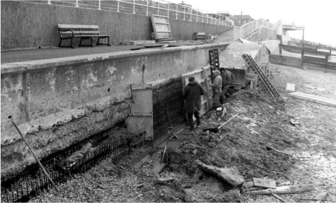
Figure 9: Underpinning a seawall affected by beach lowering at Lee-on-Solent
