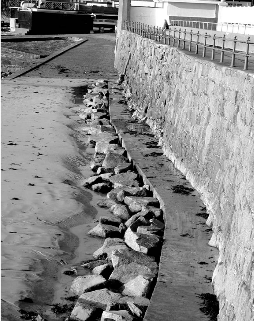
Figure 8: Mitigating scour at a seawall toe in Jersey using rock
