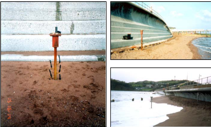
Figure 3: Monitoring scour on the beach with HR Wallingford "Tell-Tail" monitors
