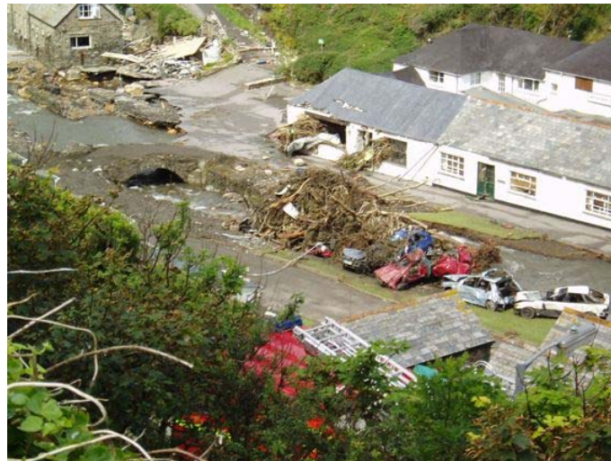
Figure 2 Flood damage at Boscastle, UK, August 2004 (Courtesy HR Wallingford)
