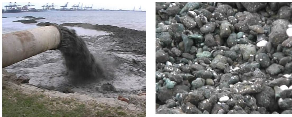
Figure 3.4 Areas 3 and 4 - Pumping clays ashore
