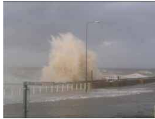
Figure 14. Overtopping at Anchorsholme, Blackpool, England on 7 December 2006 (photo by Ian Davison, Environment Agency).
