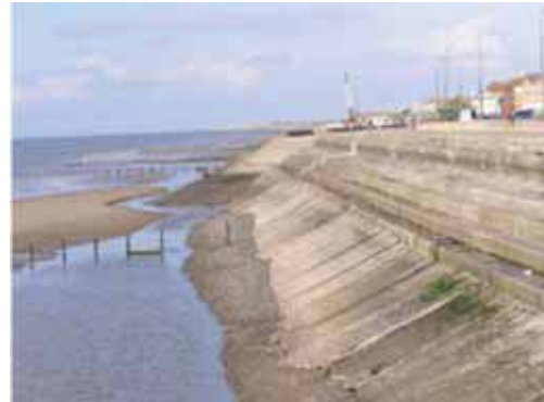
Figure 13. The seawall at Anchorsholme, Blackpool (photo by Tim Pullen, HR Wallingford).
