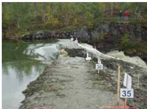
Figure 11. Converging flow dropping through a breach immediately after erosion through the upstream crest.
