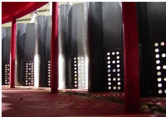
Figure 9d 16% porosity to the lower section
