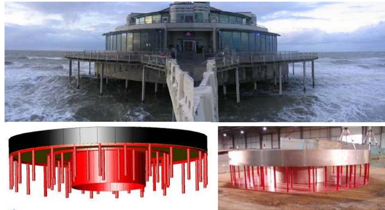
**Figure 6. Structural elements (bottom, left) and 3D physical model test set-up**
