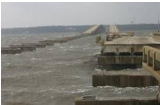
Figure 2. Wave damage to bridge decks, caused by Hurricane Katrina.
