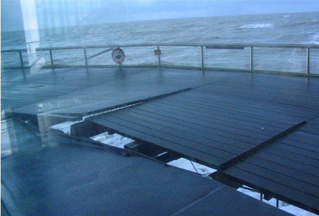
**Figure 12 Wave up-lift damage to outer walkway, 9 November 2007**
