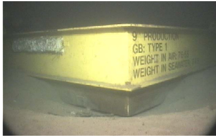
Figure 3 Small GBS in 100m of water with scour and skirt exposure (Photograph reproduced with permission from Technip Offshore UK)
