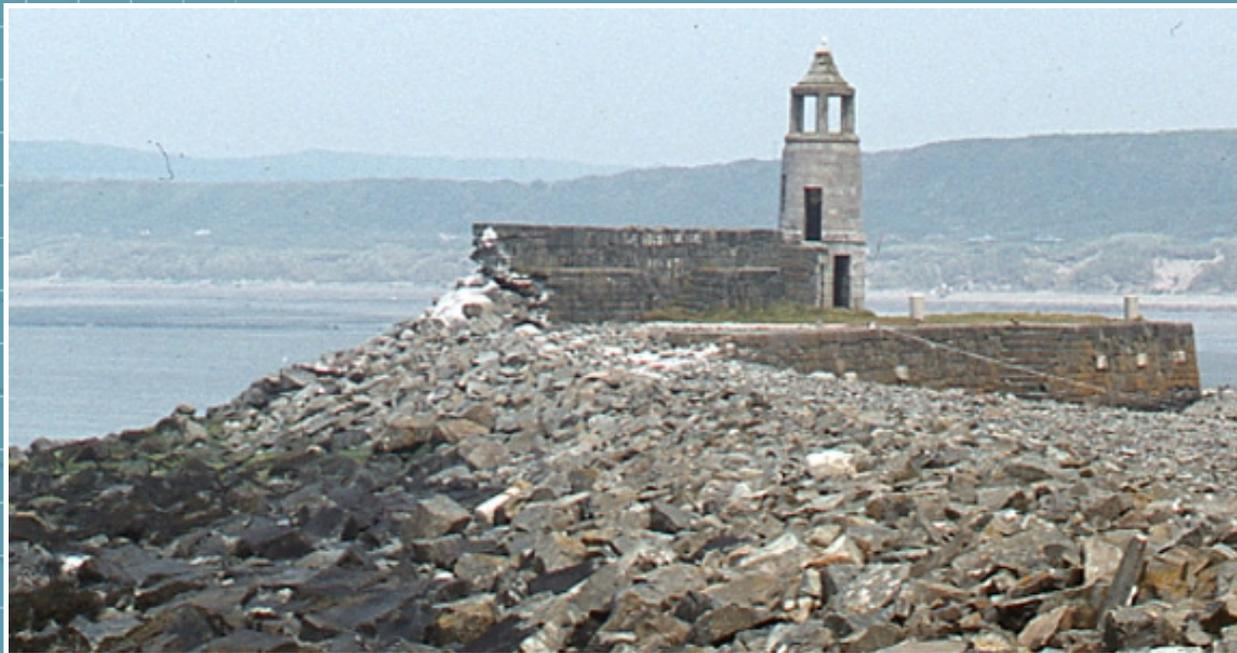
Port Logan, Rhinns of Galloway. Failure of close fitting blockwork armour (low permeability) over ungrouted rock fill.
