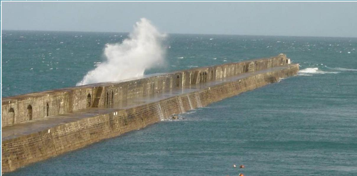
High mound causes (longer) waves to shoal up and break impulsively against the upper wave wall
