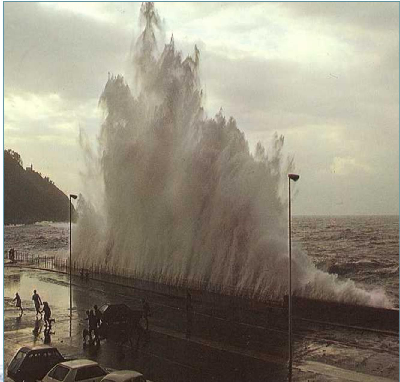
**Impulsive loads on vertical wall at Amlwch, small movements, about 1m at breakwater head.**
