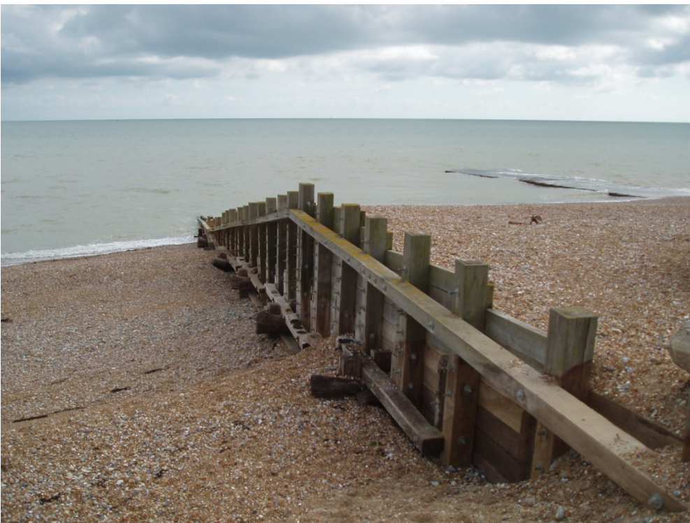
Figure 6: New groyne between Pevensey and Cooden
