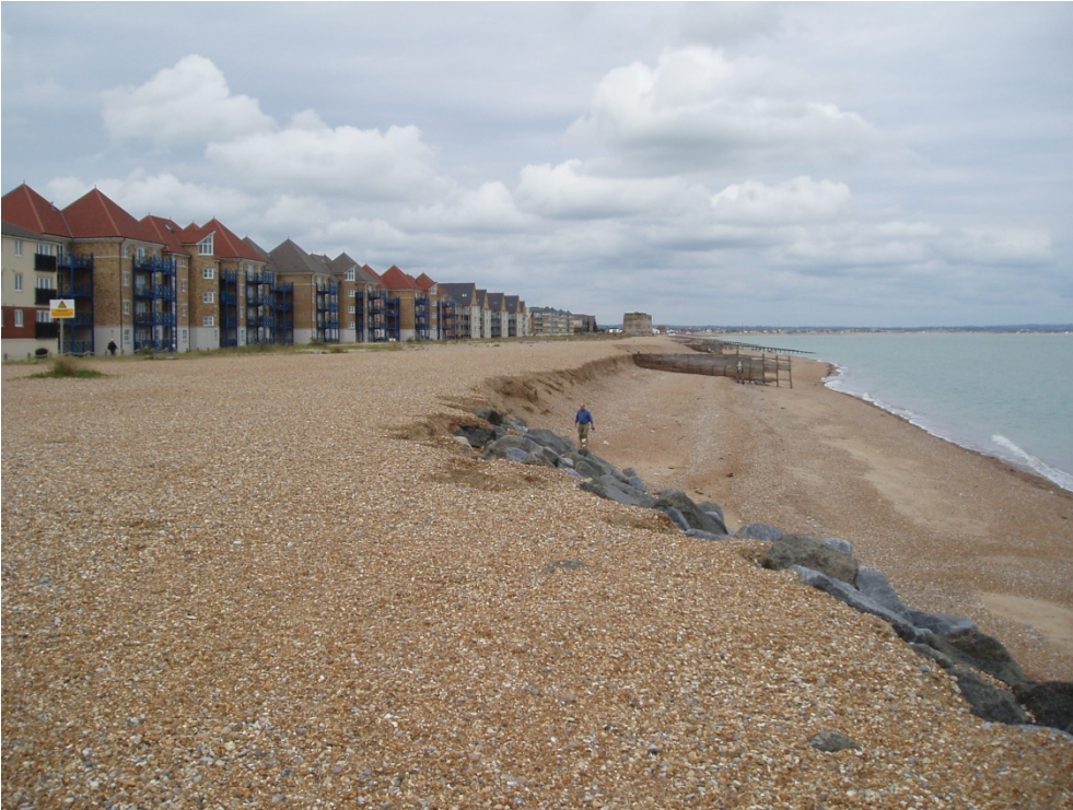
Figure 3: Erosion north of Sovereign Harbour in 2008
