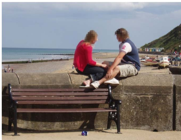
Fig. 6. Couple ‘owning’ sea wall at Cromer, UK (photo J. Simm)
