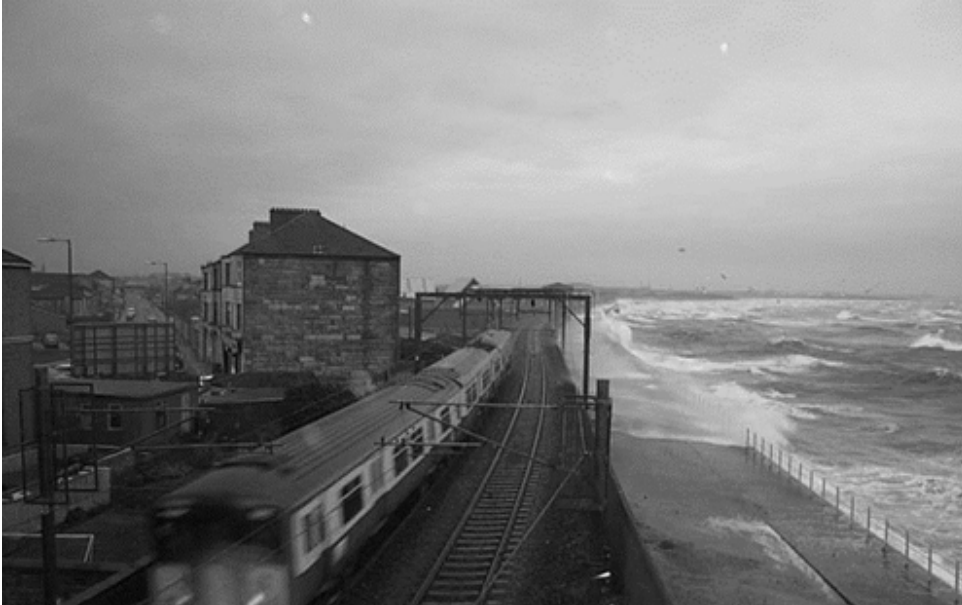
Figure 1 Rail line at Saltcoats showing heavy wave overtopping (Source Network Rail Scotland)
