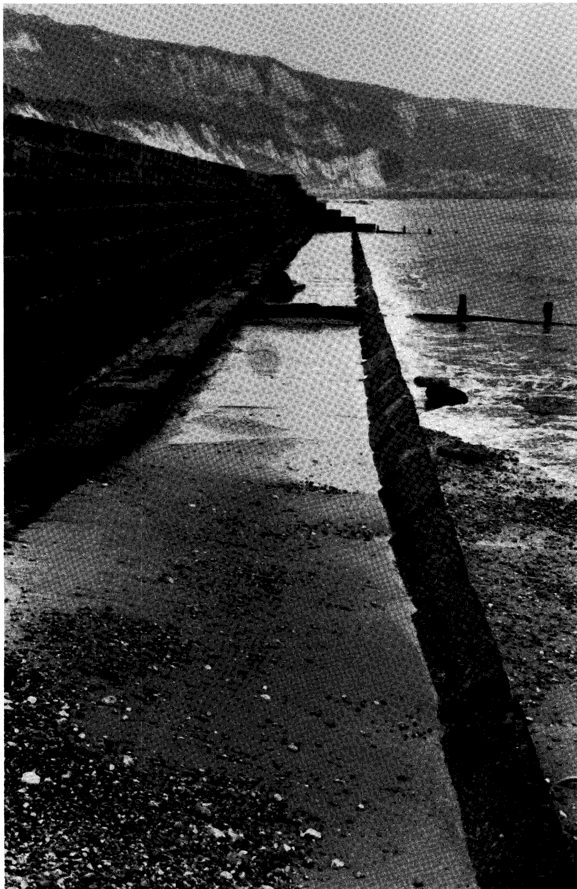
3. Sill incorporated in sea wall design, East Wear Bay, Kent
