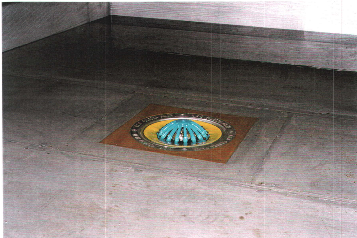
Plate 3 Outlet B with domed grating ( Q = 1.5 \text{ l/s} )
