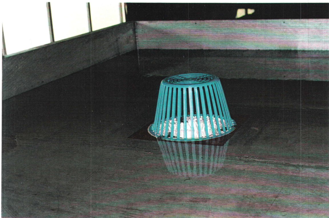
Plate 1 Outlet A ( Q = 3 \text{ l/s} )
