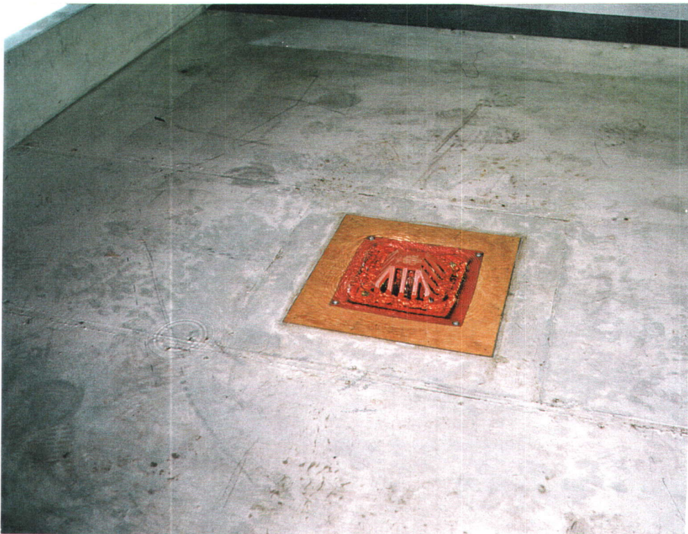
Plate 6 Outlet D ( Q = 2.0 \text{ l/s} )
