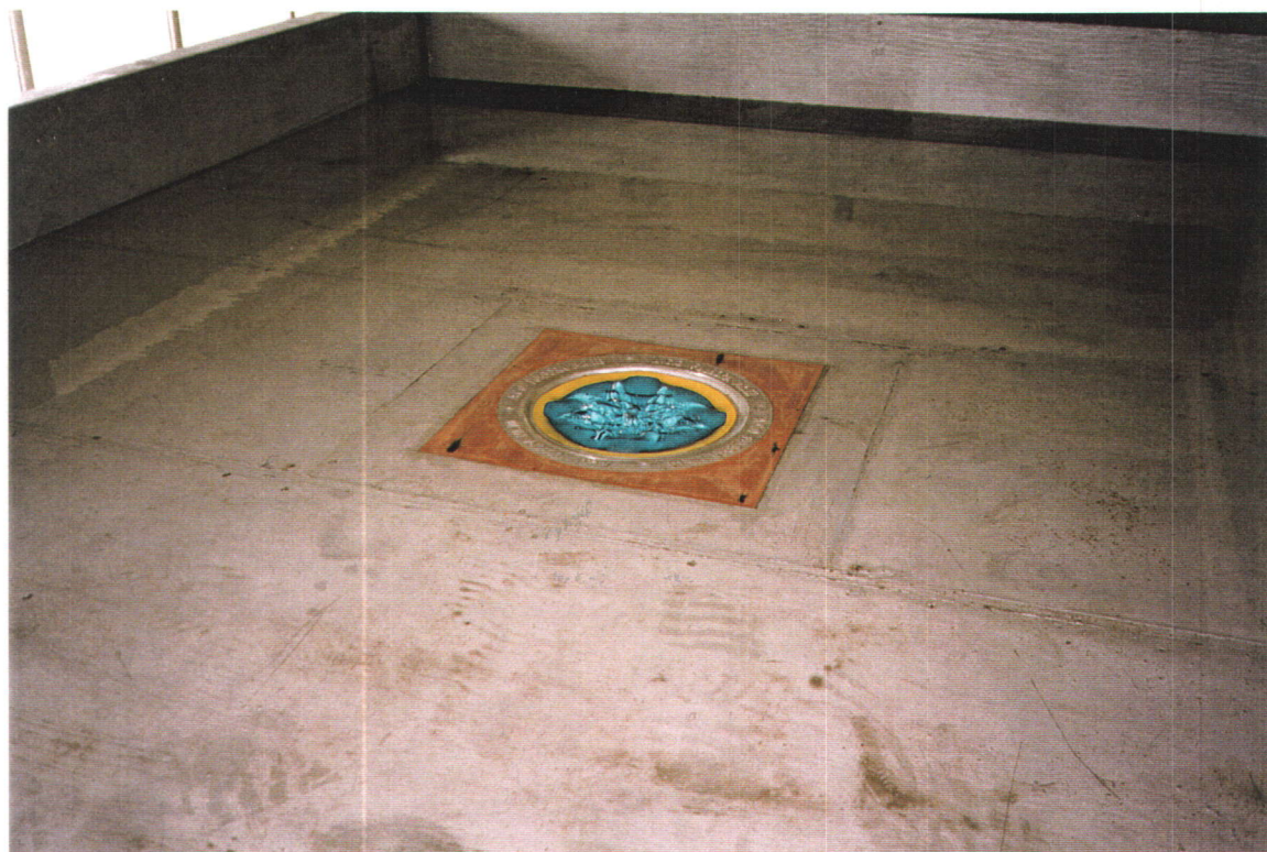
Plate 4 Outlet B with flat grating ( Q = 3.4 \text{ l/s} )
