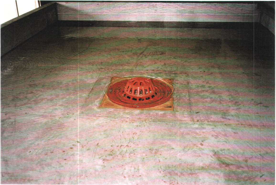
Plate 5 Outlet C ( Q = 6.1 \text{ l/s} )
