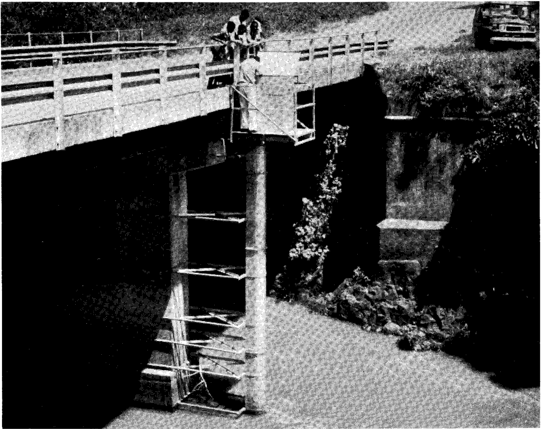
Plate 1 Partech meter housing at site 4BC2
