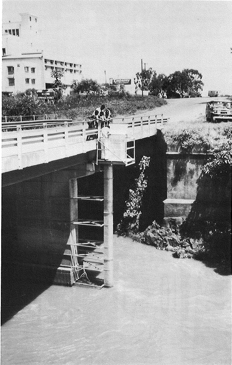
PLATE 1. Partech installation at Sagana Bridge
